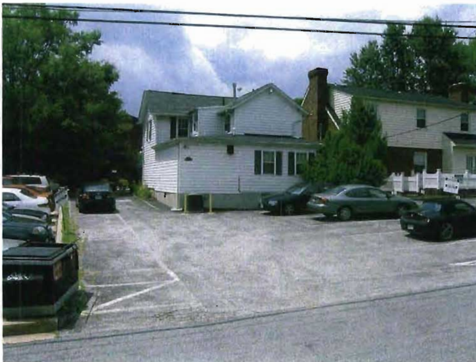
Existing Structure, Looking West from Alley
