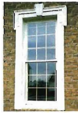
Windows, w/ accentuated detailing
