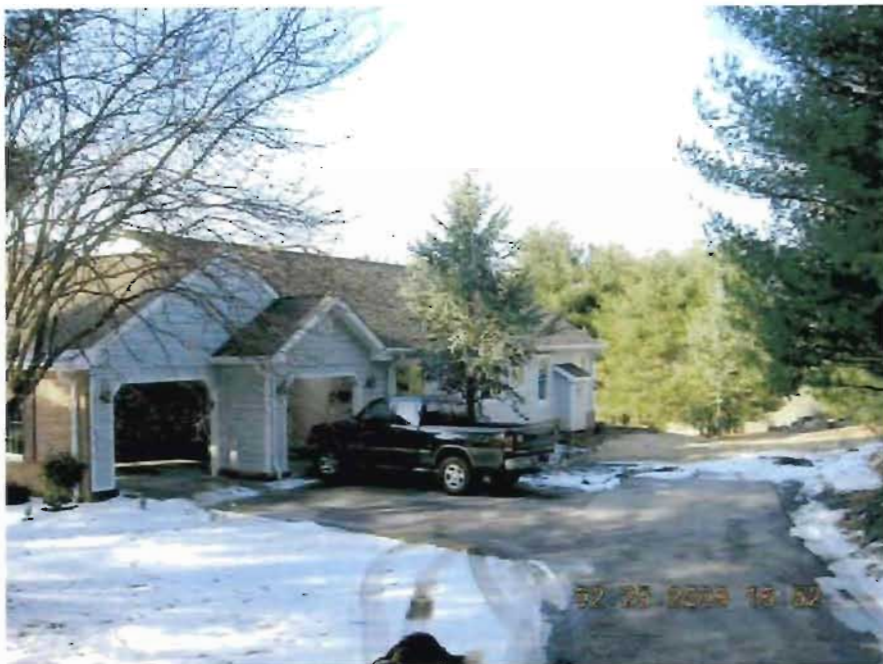
RIGHT (EAST) ELEVATION SHOWING ORIGINAL GARAGE AND NEW ADDITION
