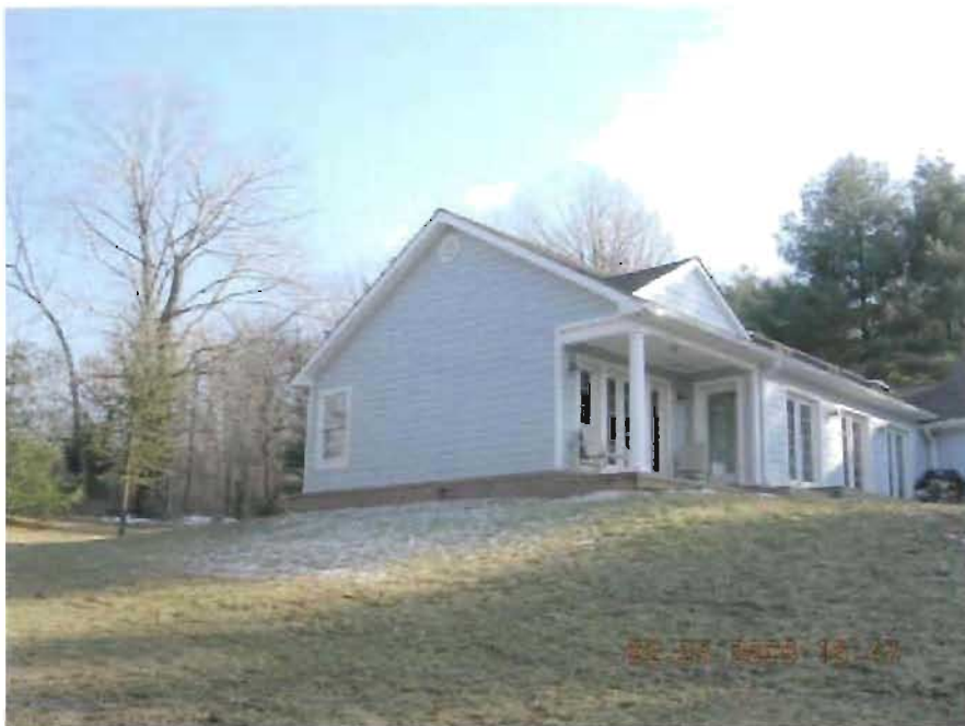
REAR (NORTH) ELEVATION OF ADDITION
