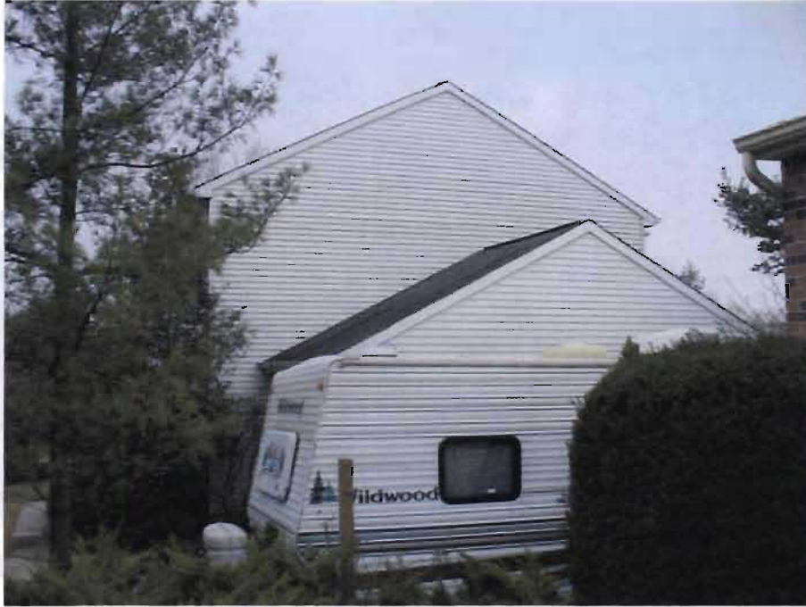
Looking at the side of 1 Hurstoak Court
