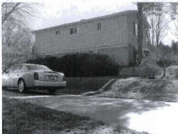
View of 4600 Hawksbury Rd. *windows*
