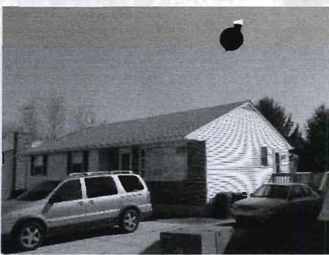
View of neighbor at 9476 Seven Courts Rd *Window and door*
