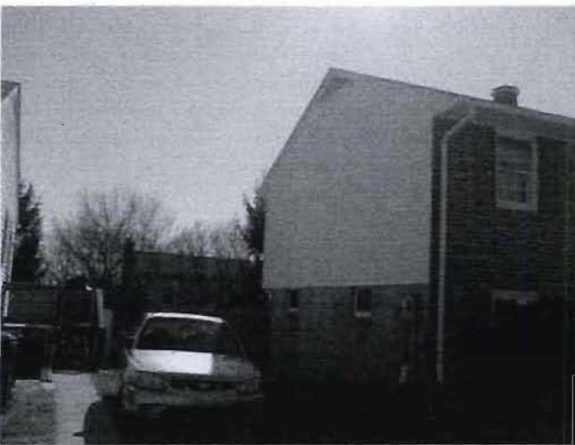
View of north side of house *basement windows*
