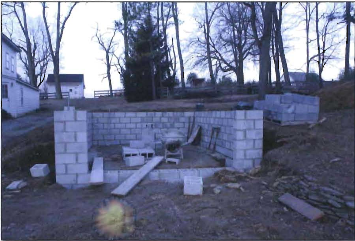
IMG 4 – Progress as of 3/13/08
