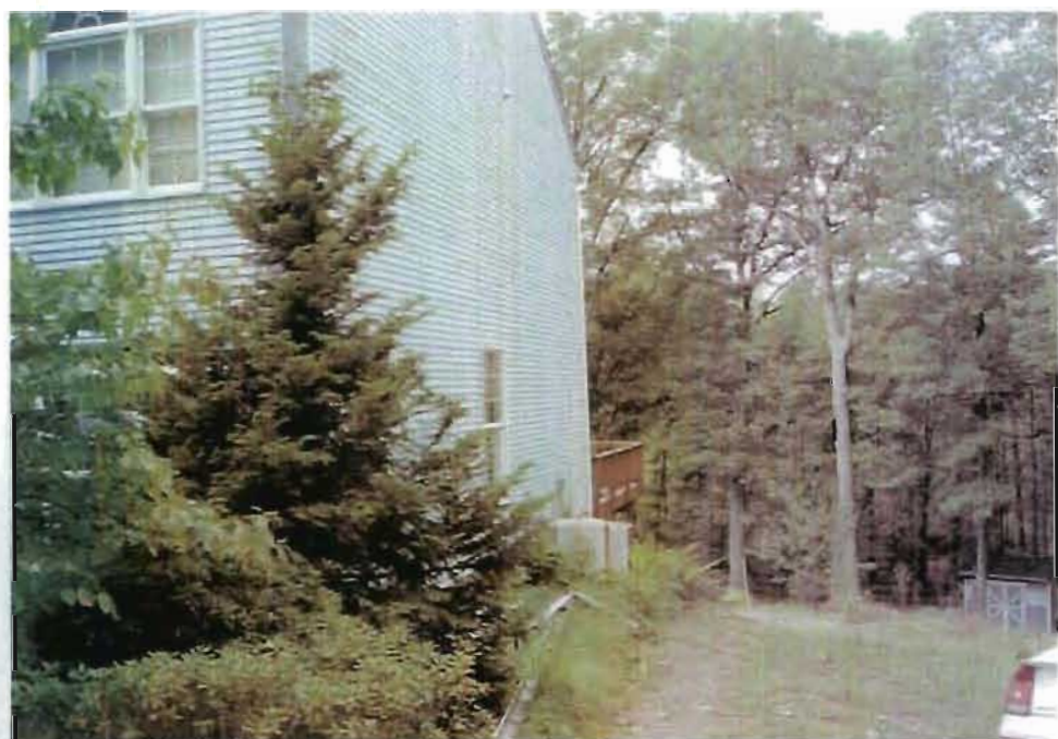
LOOKING FROM FRONT ON SIDE OF BUILDING. CLOSE
