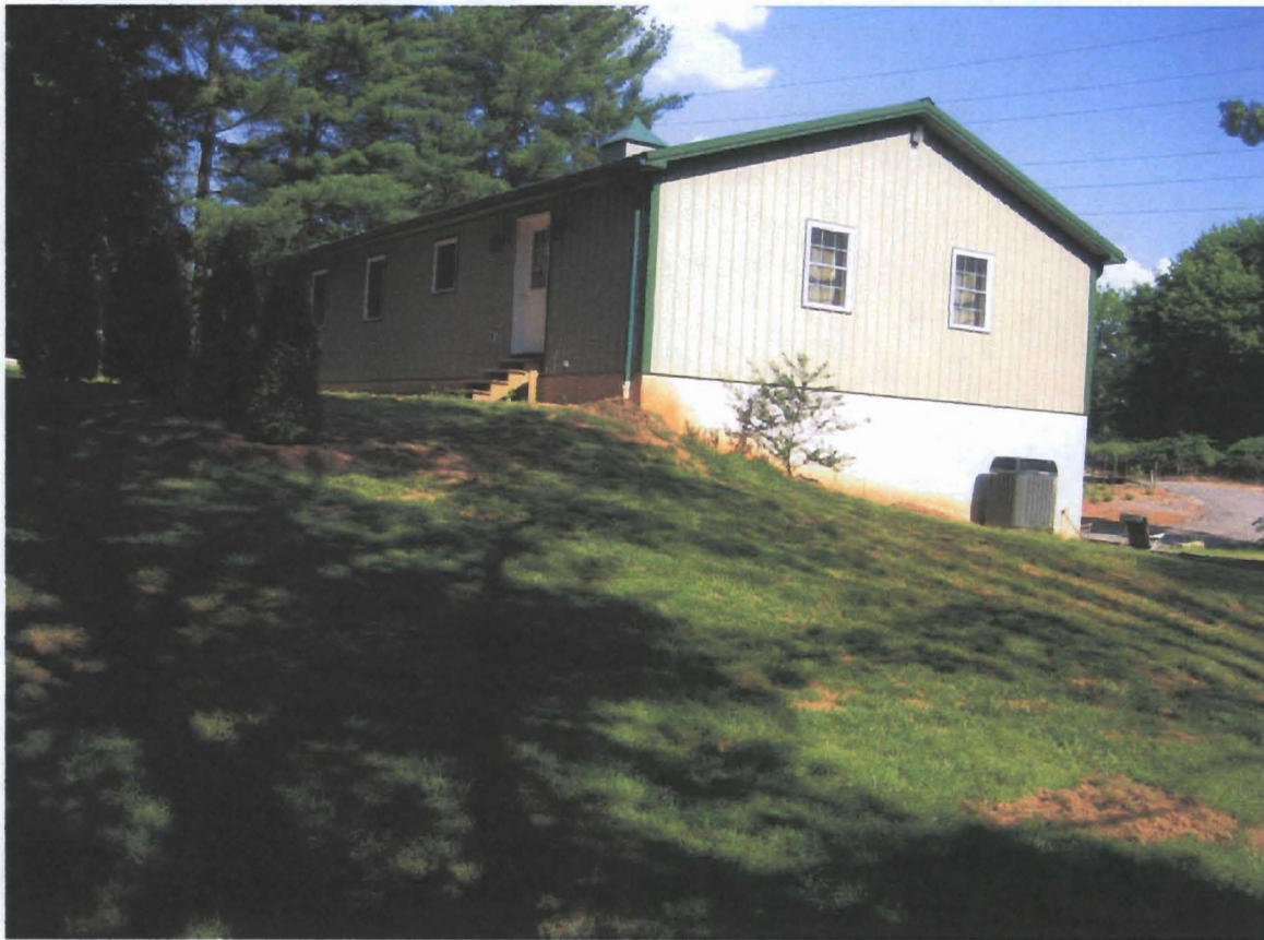
EXTERIOR GRADE ARTIFICIALLY BUILT UP – 15' HT. EXCEEDED
