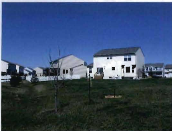
3 CORAL CT. REAR OF HOUSE (FACING NORTH)
