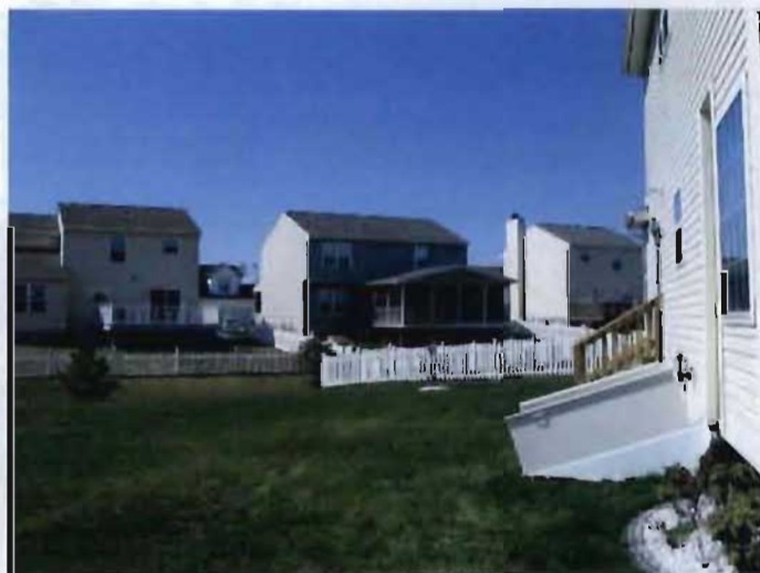
3 CORAL CT. REAR OF HOUSE (FACING WEST)
