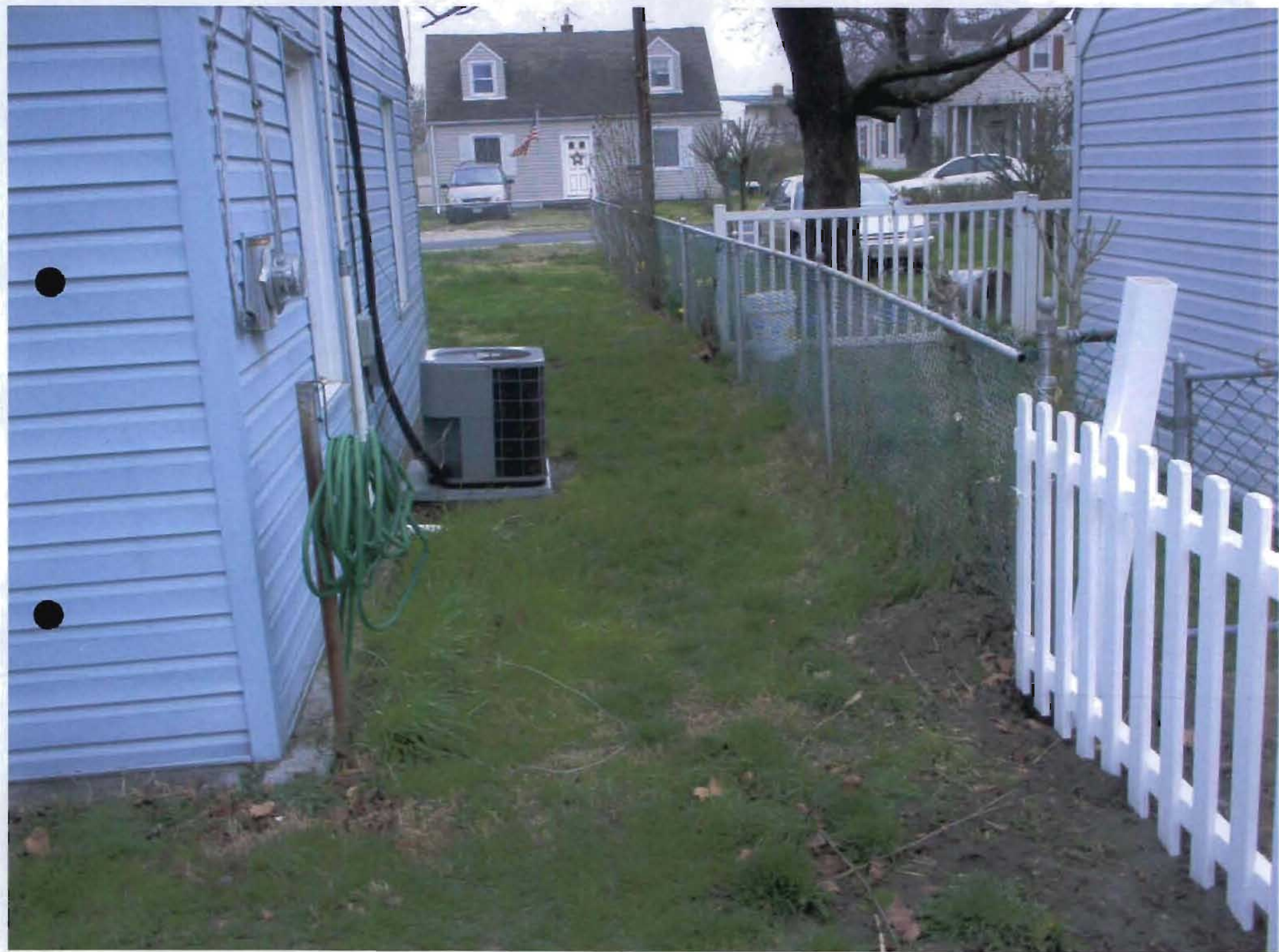
Wetr Side of house 3421 Sollers Point Road
