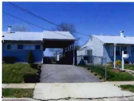
Carport @ side yard
