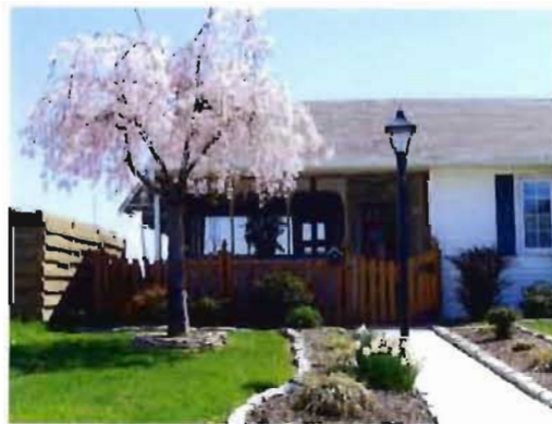
Roofed porch @ side yard
