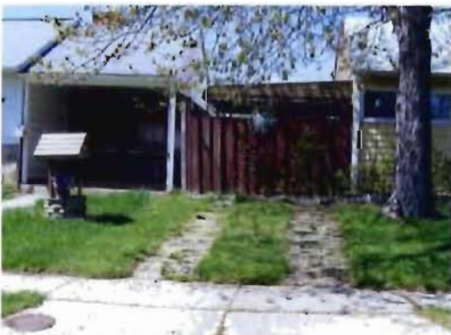
Dwelling & porch @ side yard
