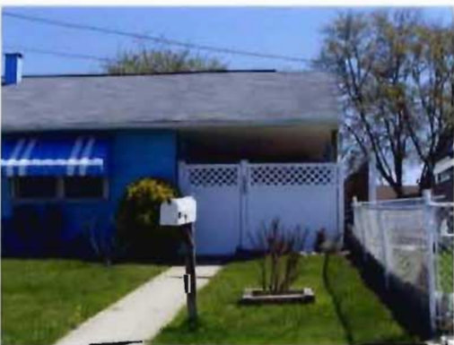
Dwelling & porch @ side yard
