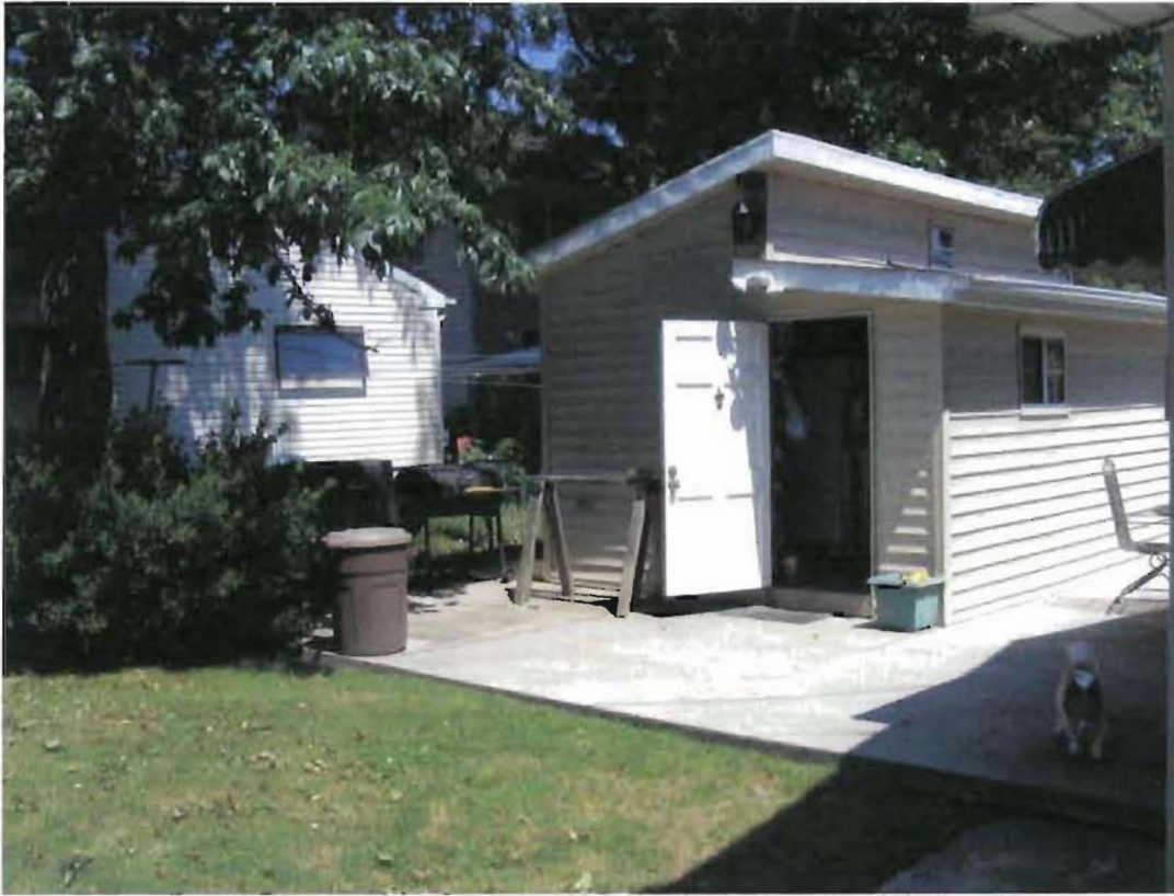
NW CORNER OF DWELLING LOOKING EAST TOWARD SHED
