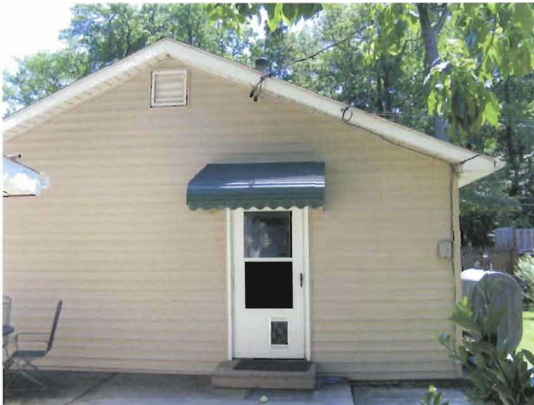
REAR OF PROPERTY LOOKING TOWARD REAR OF DWELLING
