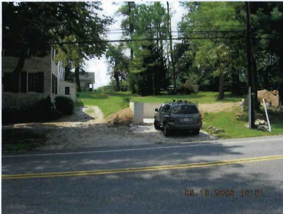
GARAGE UNDER CONSTRUCTION AT #21010 YORK ROAD, RIVERA RESIDENCE
