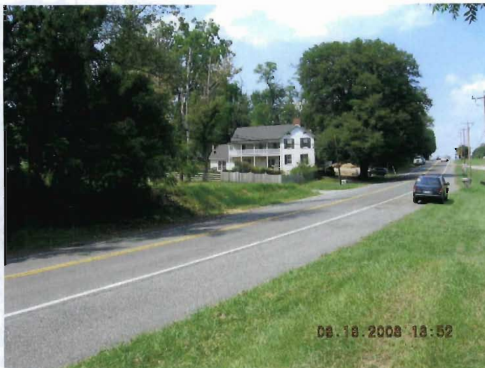
VIEW FROM CENTER OF SITE TOWARDS #21010 YORK ROAD, RIVERA RESIDENCE
