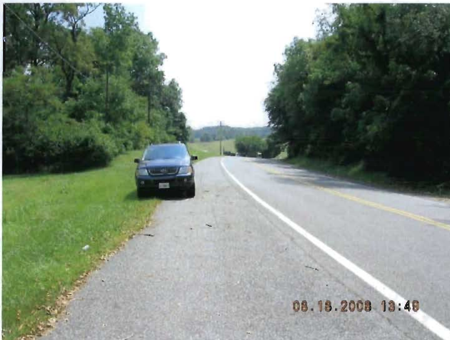
LOOKING SOUTH ALONG YORK ROAD FROM PROPOSED DRIVEWAY LOCATION
