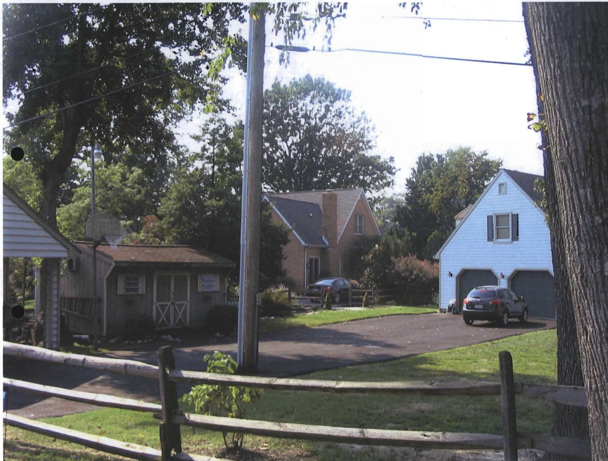
Adjacent Dwelling Garage and Other South Dwelling
