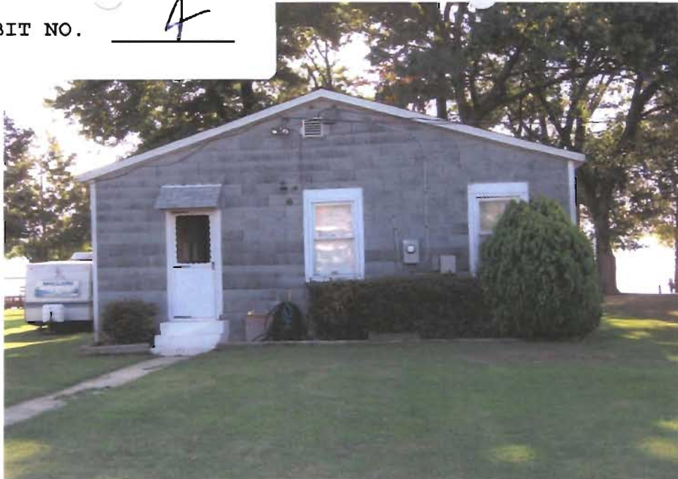
1332 E. RIVERSIDE EXISTING STRUCTURE FROM ROAD
