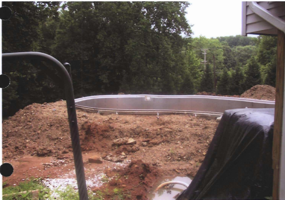
View from Basement Door
