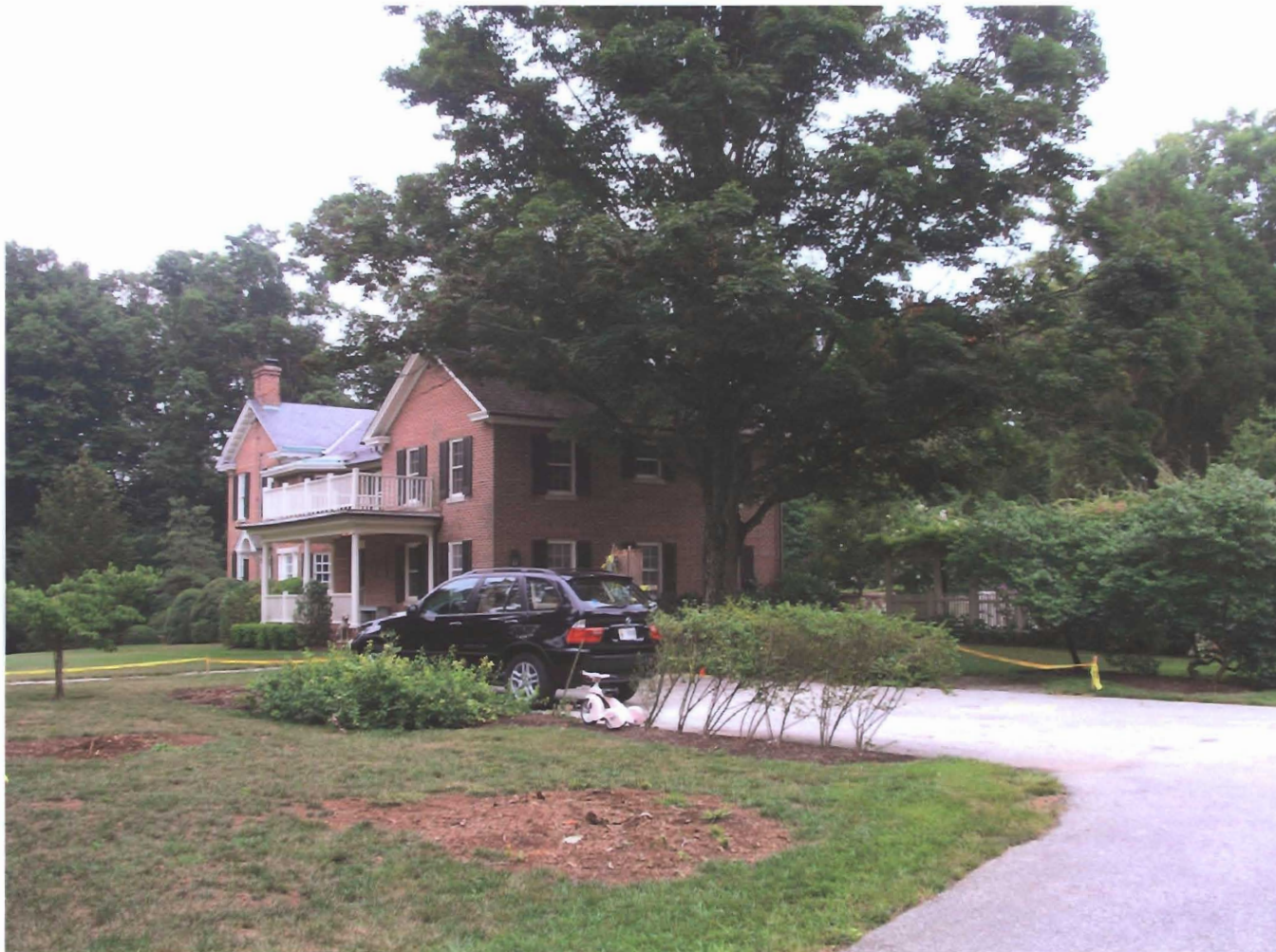
Site of proposed garage in back yard
