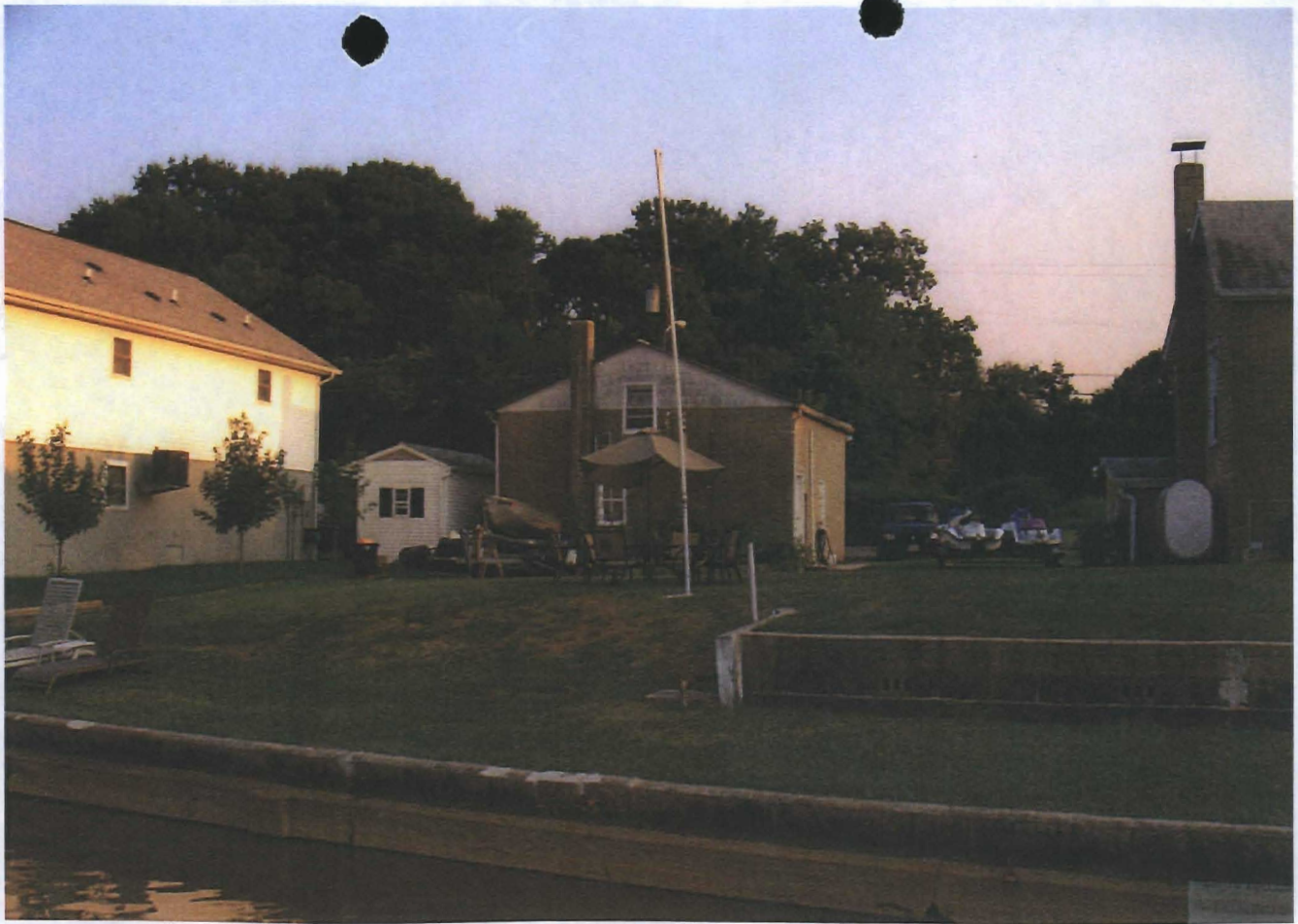
8. McCormack Garage and Storage Building , looking toward Horne Residence and shed form pier.
