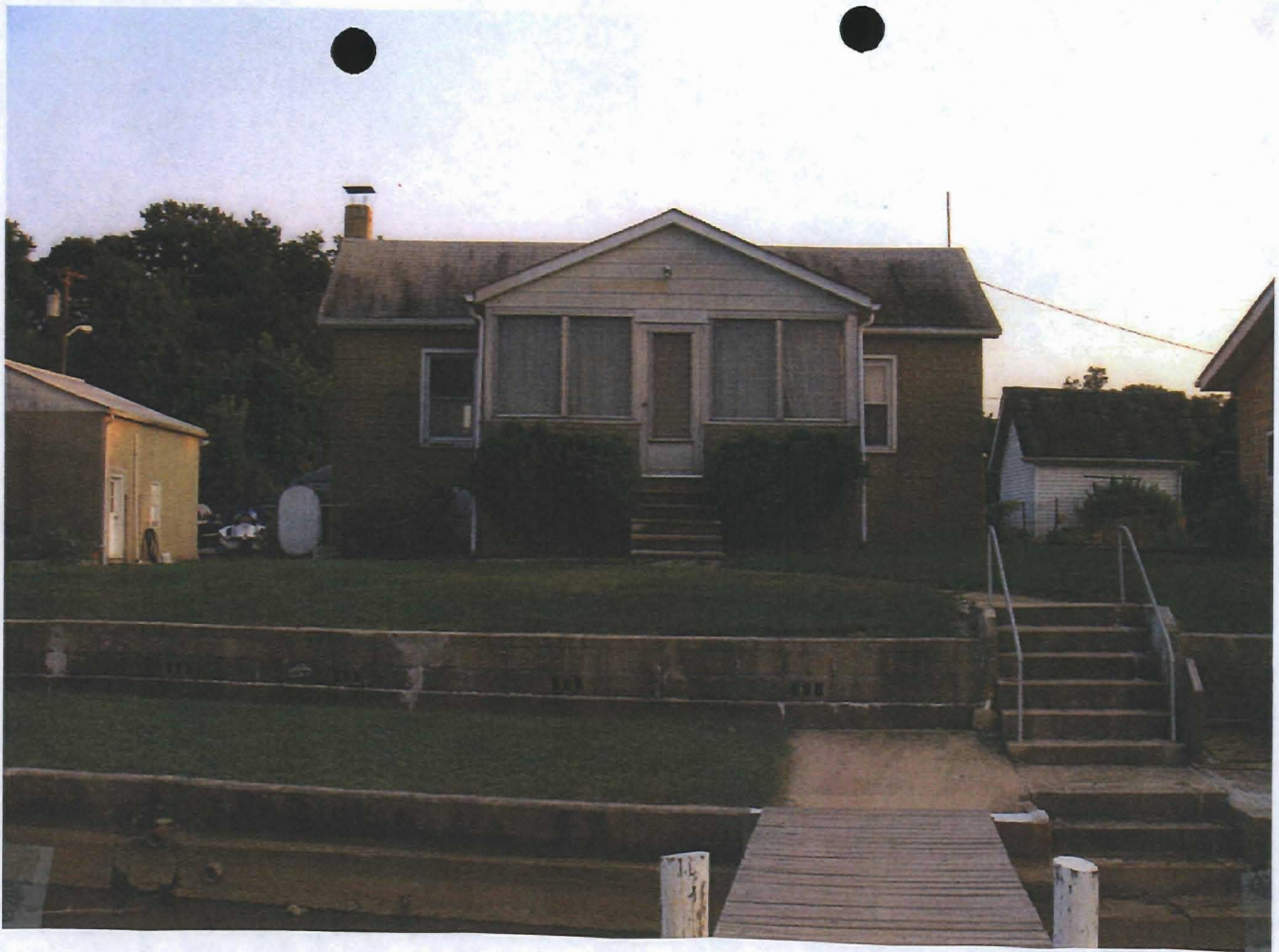
4. North waterside facade of McCormack Residence from pier.
