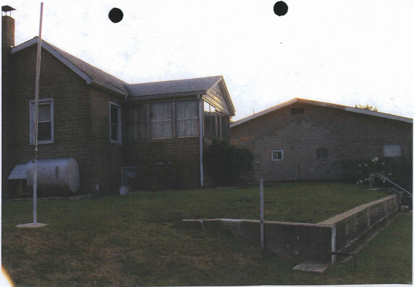
6. McCormack Residence taken from eastern end of bulkhead looking at Retaining Wall and Wasilewski Residence.
