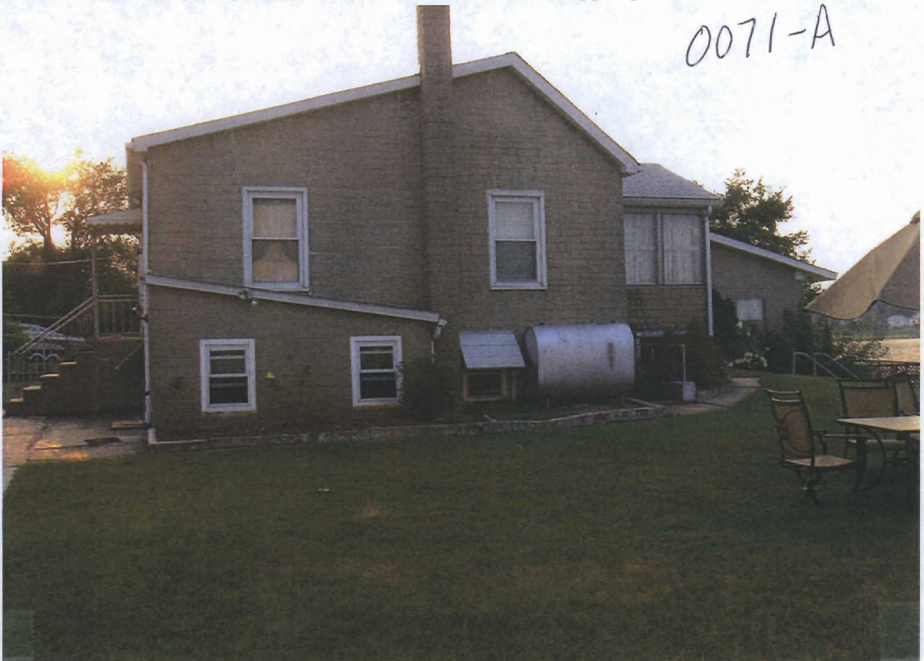
3. East facade of McCormack Residence
