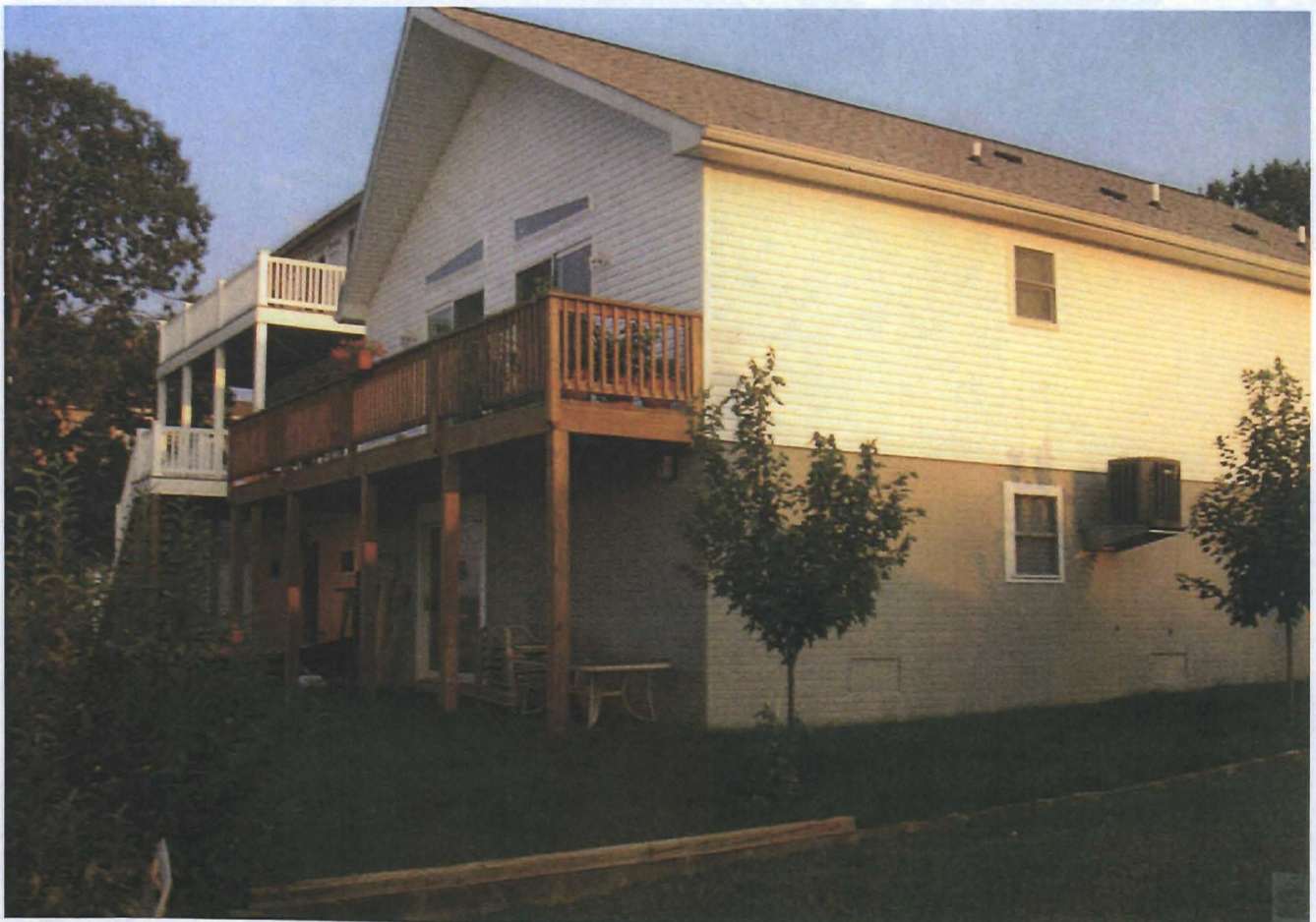
7. Horne Residence at 11226 Bird River Grove Road.
