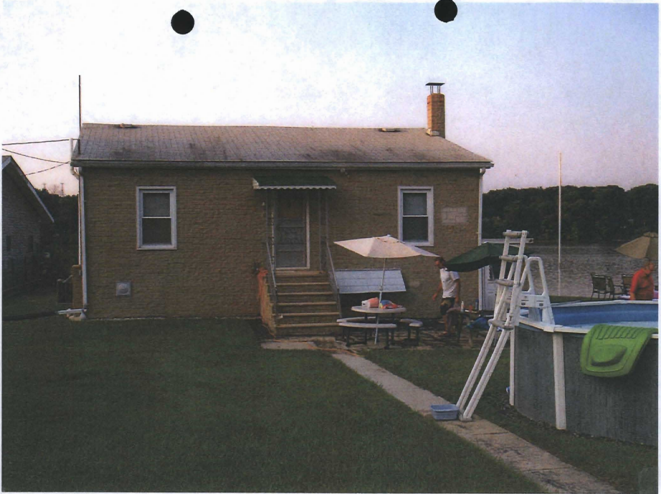
2. Roadside (South) facade of McCormack Residence, looking past pool.
