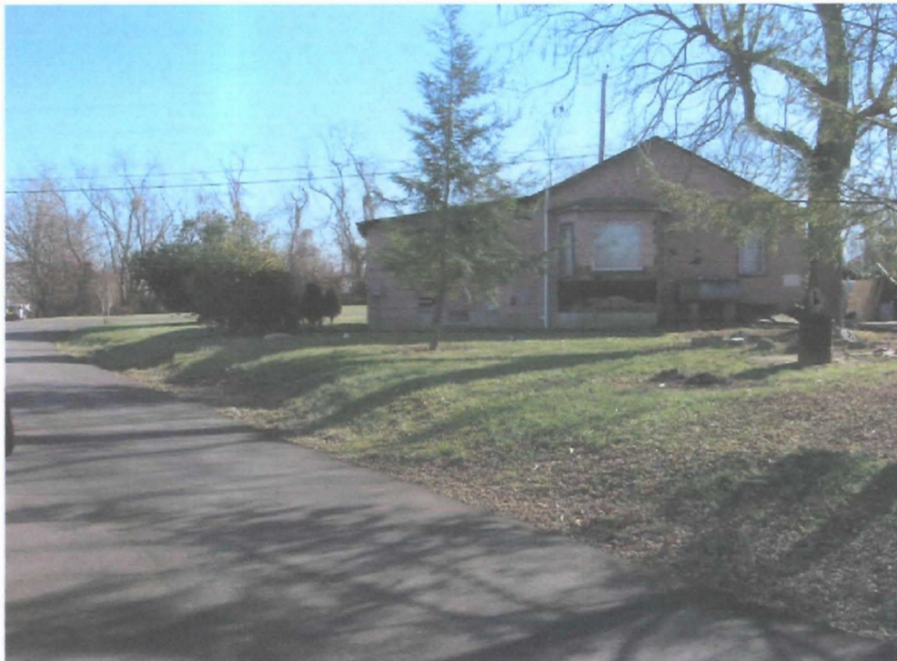
REAR ELEVATION OF #257 HENRIETTA AVENUE
