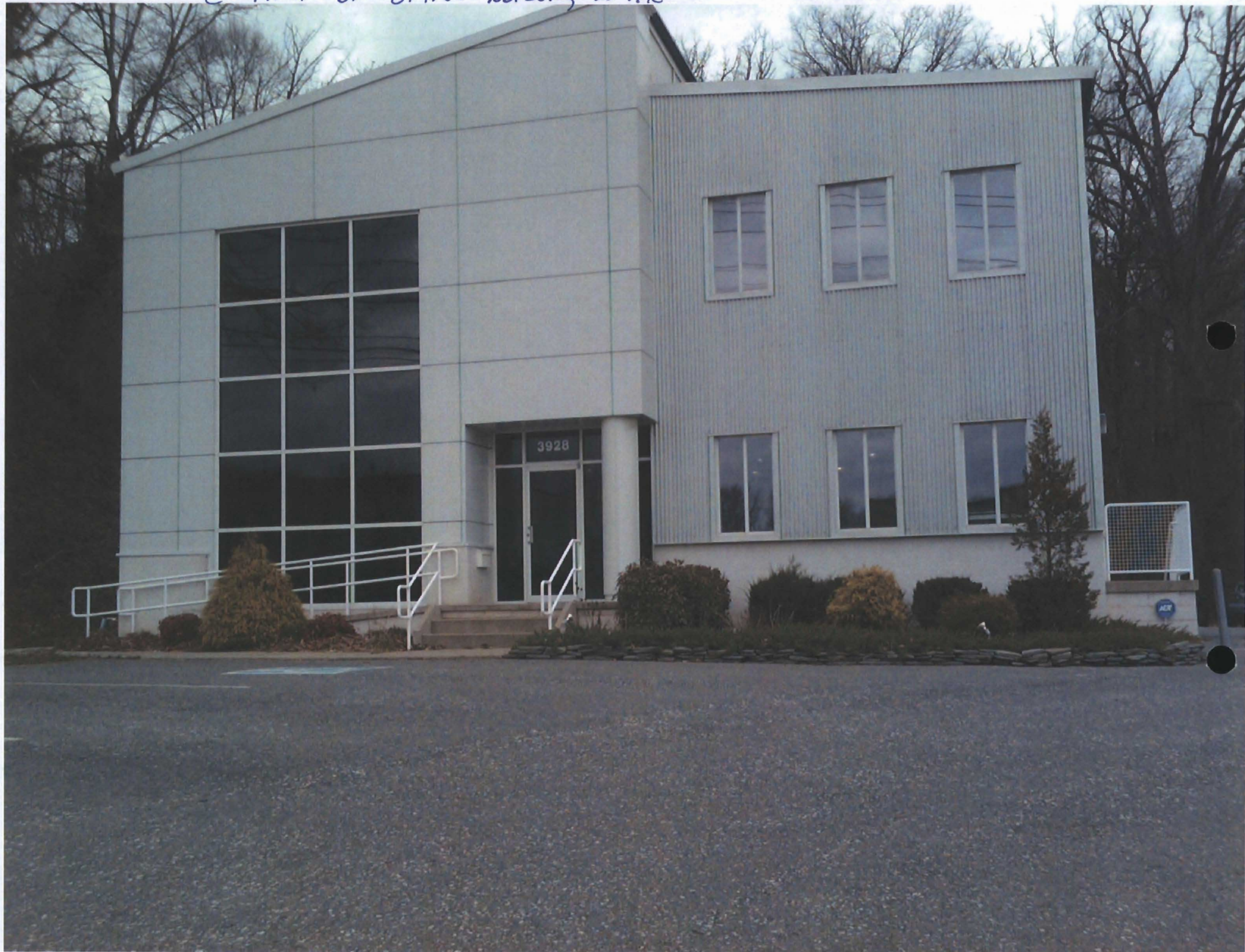
C- FRONT OF OFFICE BUILDING ON SITE
