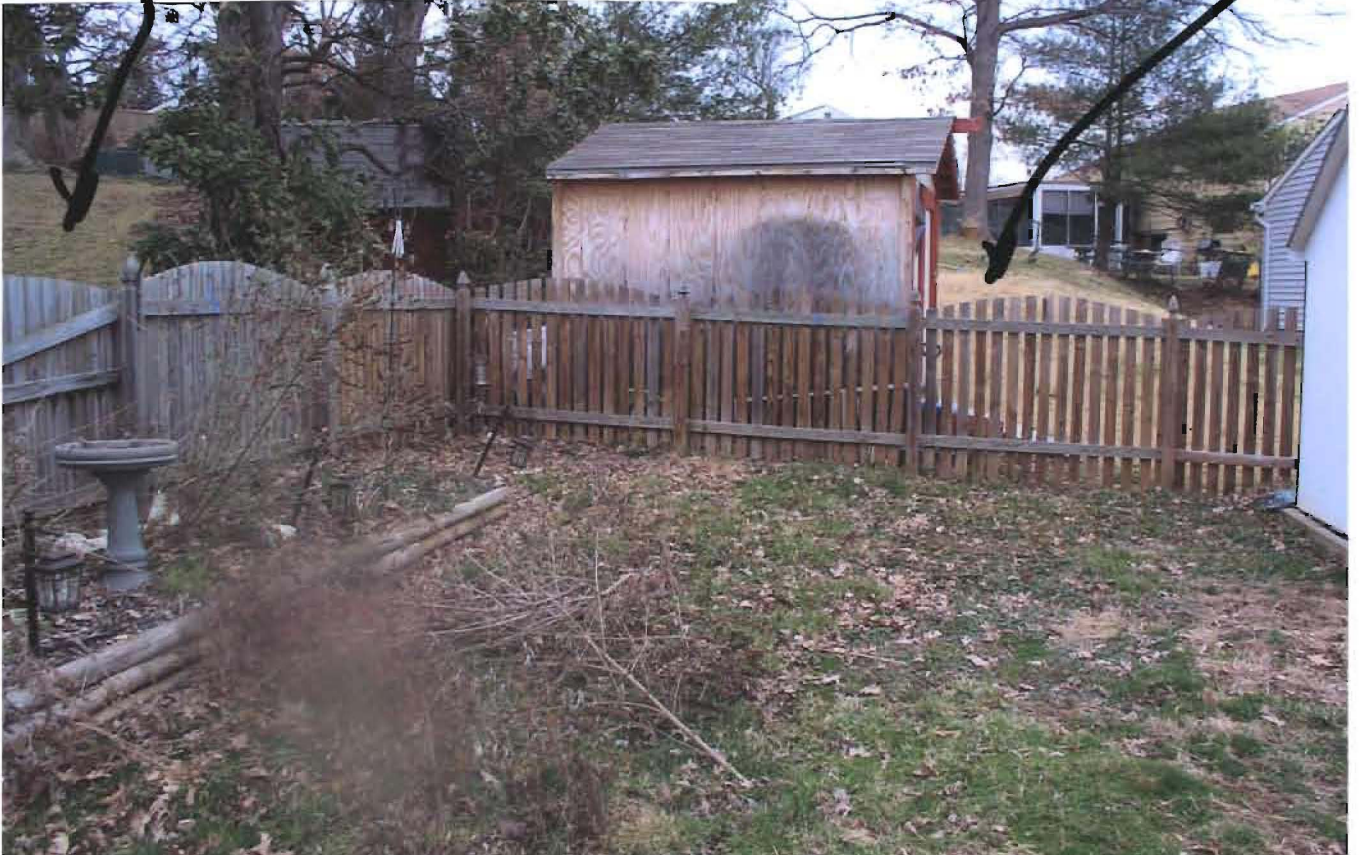
WATER RUN OFF FROM 2 HILLS BEHIND 1202 ROBIN CT. (WEST OF 5724 OAKLAND ROAD)
