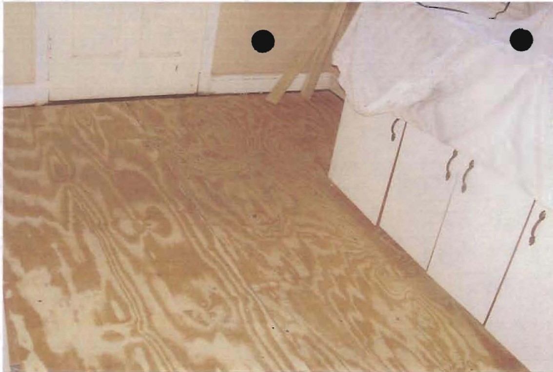
1st Floor Apt. Kitchen New sub floor Ex 11
