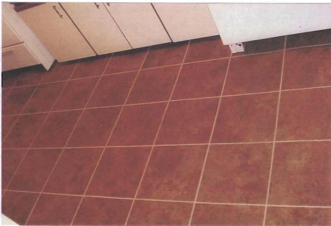
1st Floor Apt. Kitchen - New Flooring (Present)
