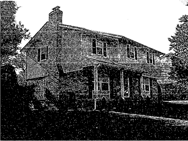
Front Veiw of our property 212 Wickersham Way
