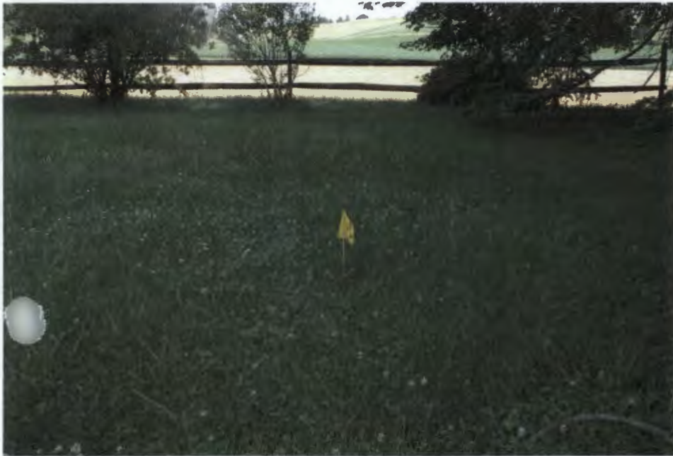
1. Looking south. Flag is location of far corner of addition.
