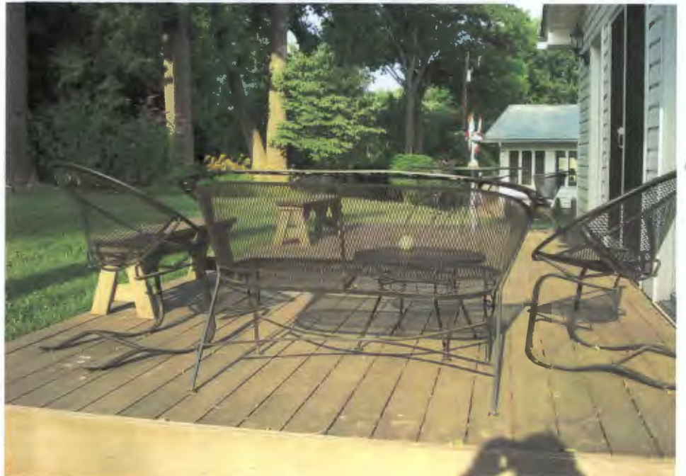
EXISTING DECK TO 924 BREZEWICK CIRCLE
