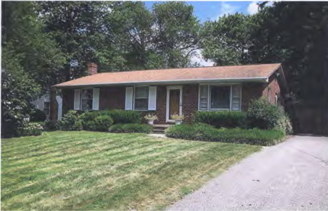
Front elevation and Driveway at 1617 as viewed from the street
