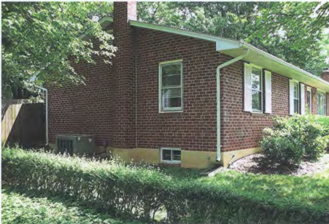
West Side elevation of 1617 as viewed from 1703
