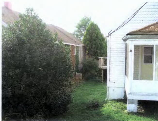
View of area between buildings on 2342 (right) and 2340 (left) York Road Properties. View is from sidewalk along York Road. Area of proposed connection between buildings.
