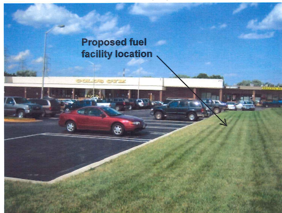
Another view of the proposed fuel facility location.
