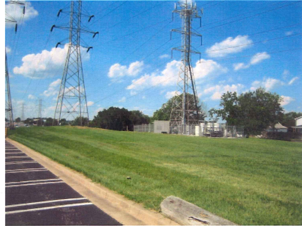
View of electric transmission wires to the east.
