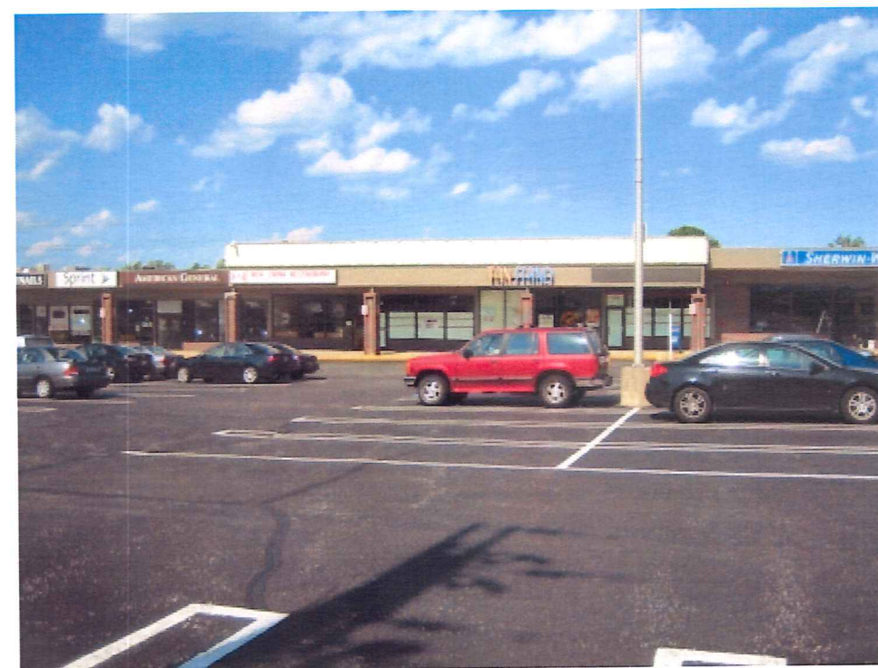
Additional views of the shopping center looking east.
