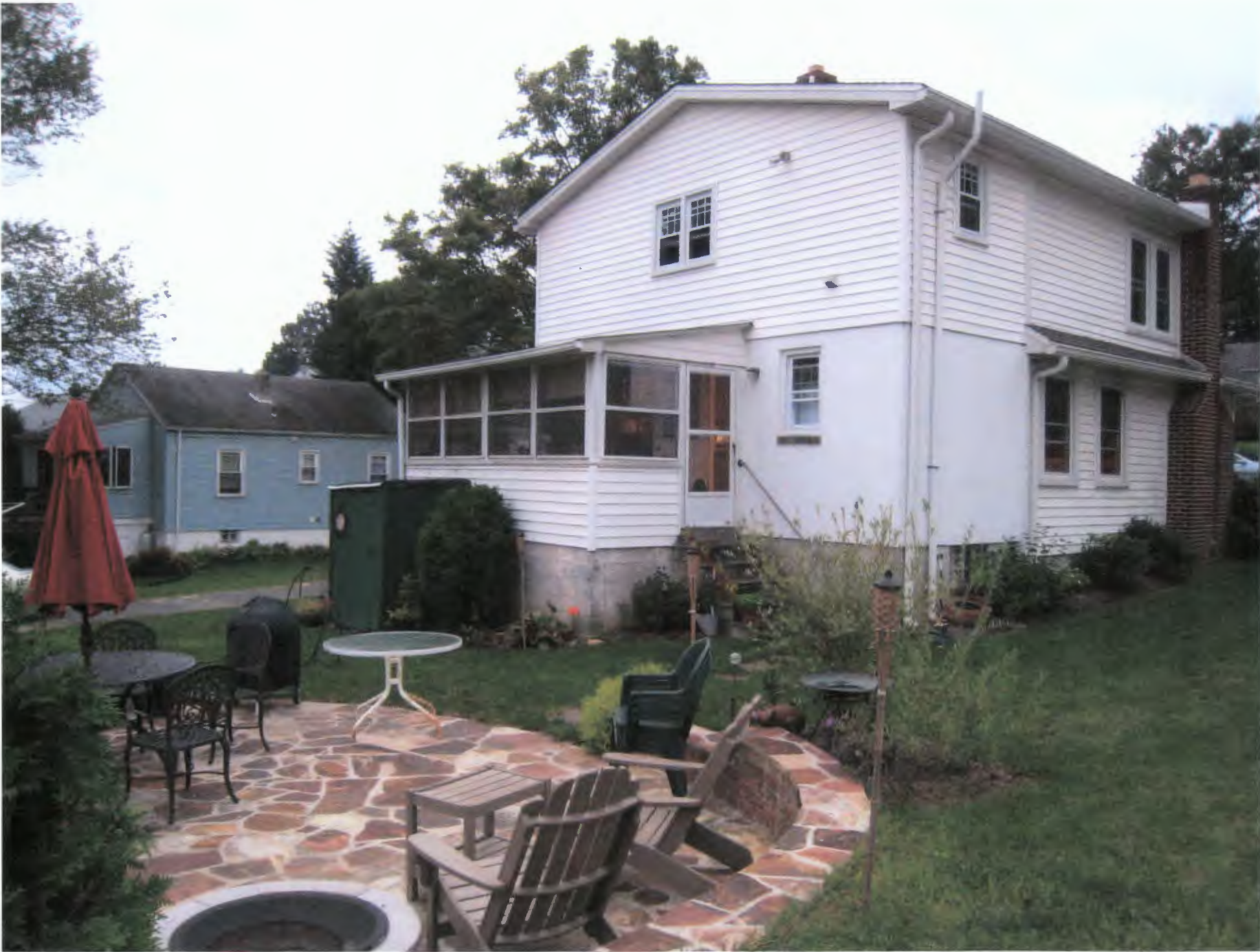
Backyard from left side, rear of property (from street)
