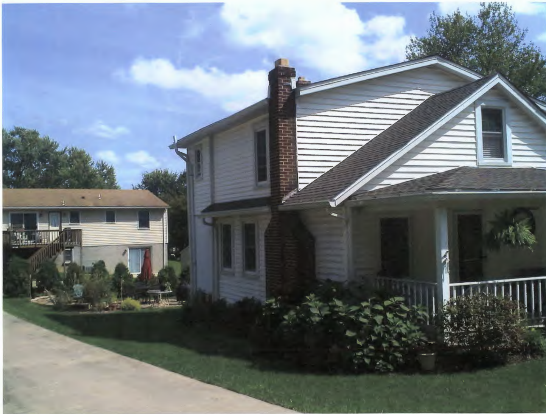
Front & left of House, showing rear yard & rear Neighbors house.
