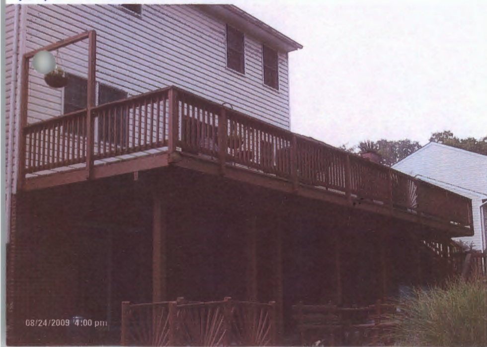
Right side of property rear view
