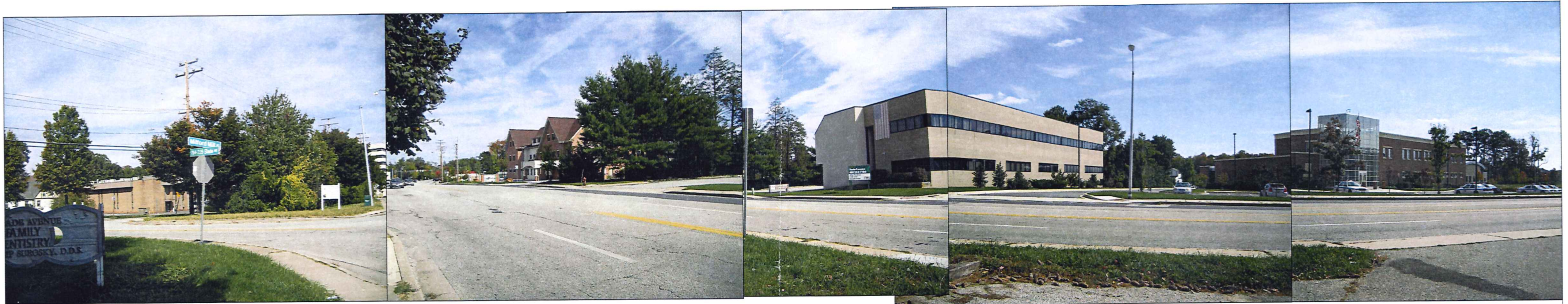
ELEVATION OF MILLFORD ROAD (across the street)
