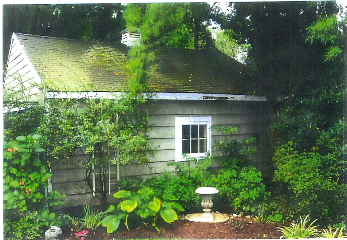
Existing Garage, WEST side:
