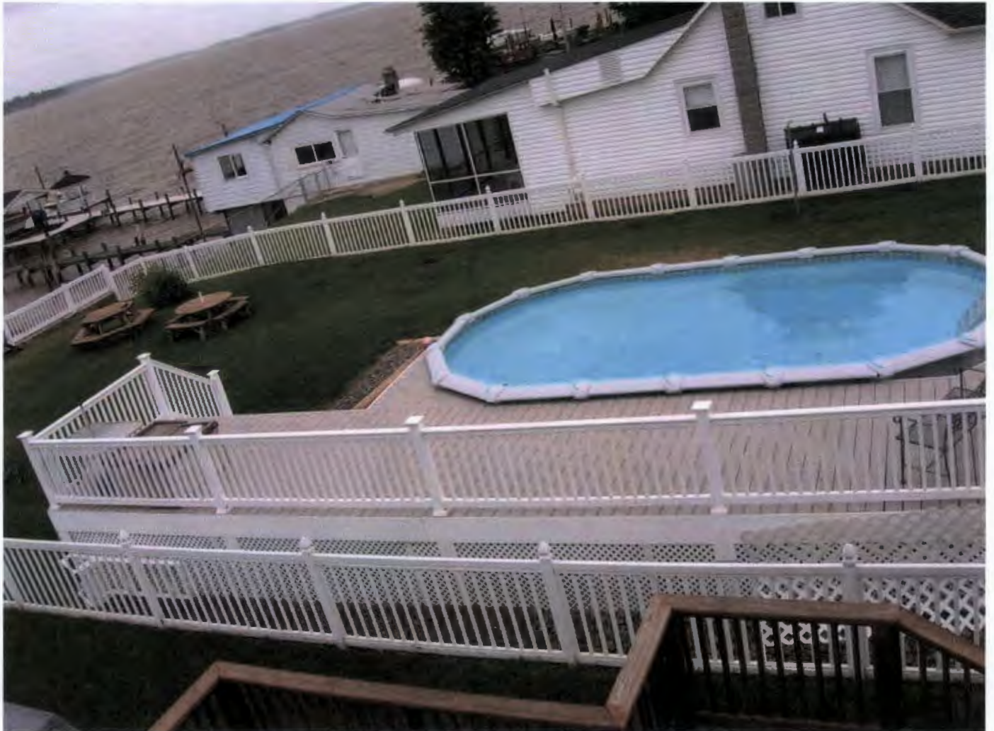
View of Ms. Treat's existing deck and pool: Both built without permits and 19 inches off property line.
