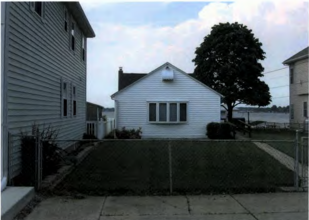
View of Sullivan's yard: Fire code violation to have two buildings so close together?
