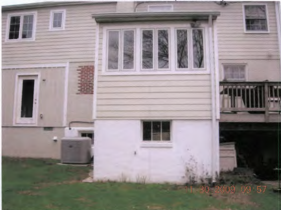
REAR OF EXISTING DWELLING, IN AREA OF PROPOSED 1-STORY ADDITION
