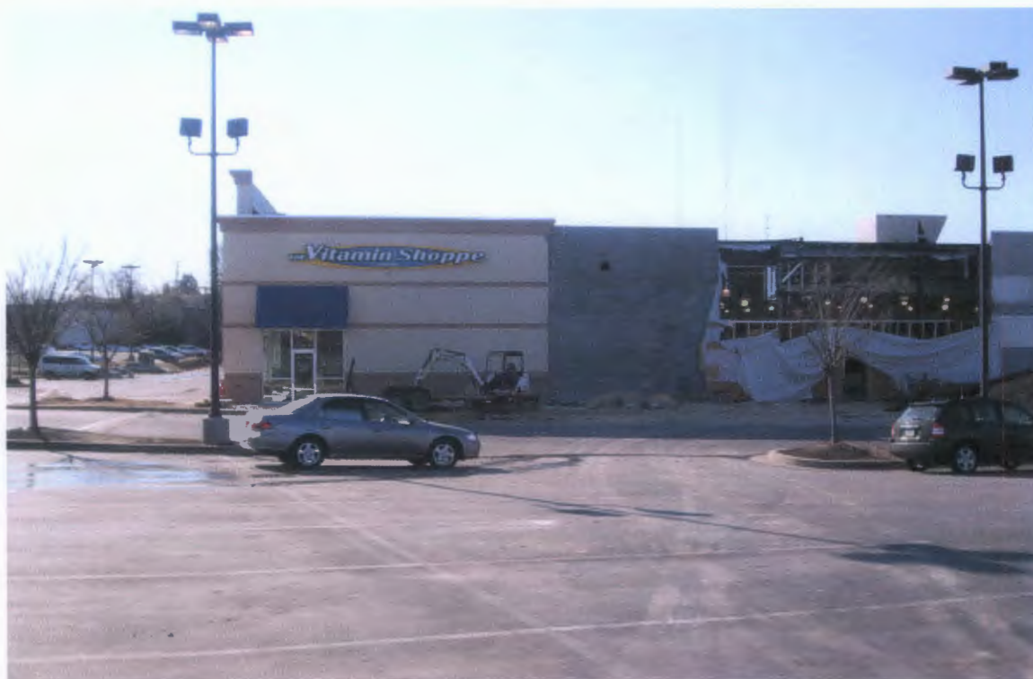
Front of HHGregg store (east side of building)
