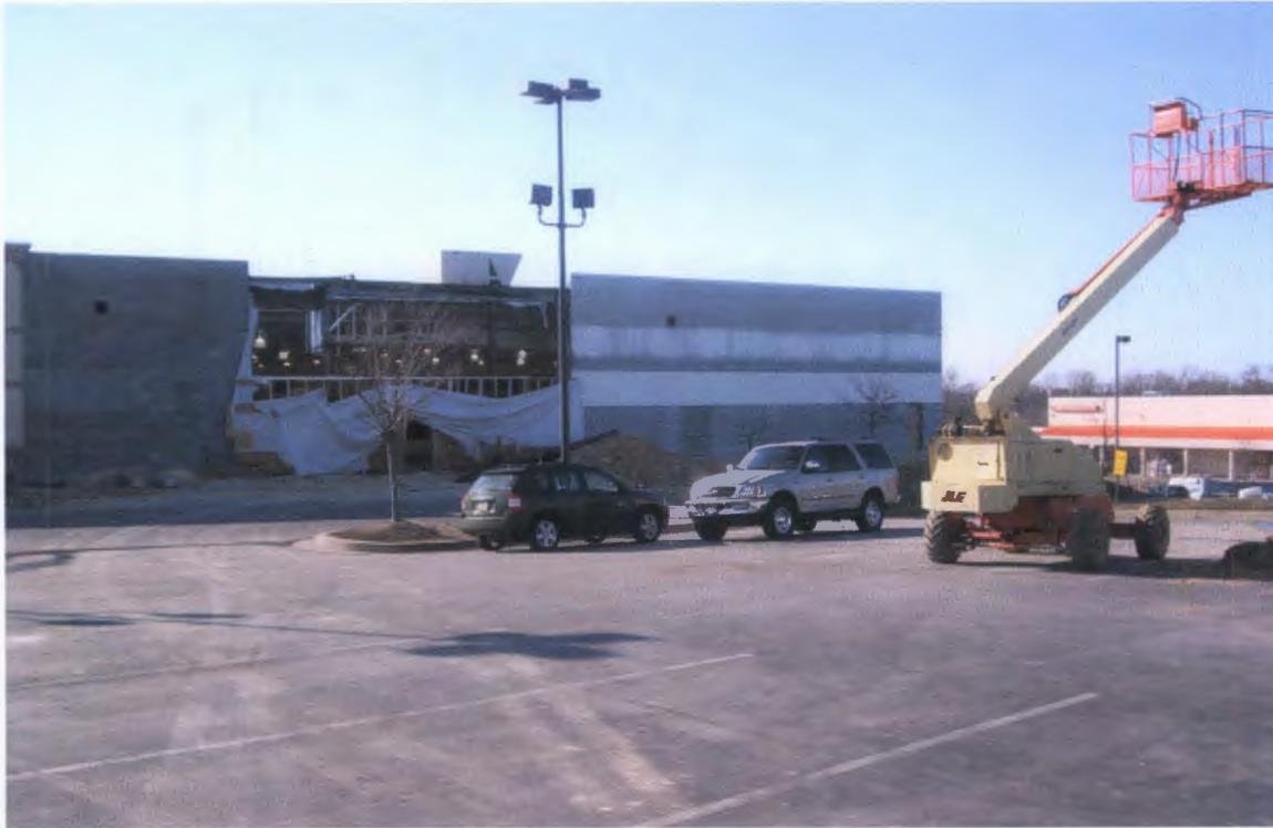
Front of HHGregg store (east side of building)
