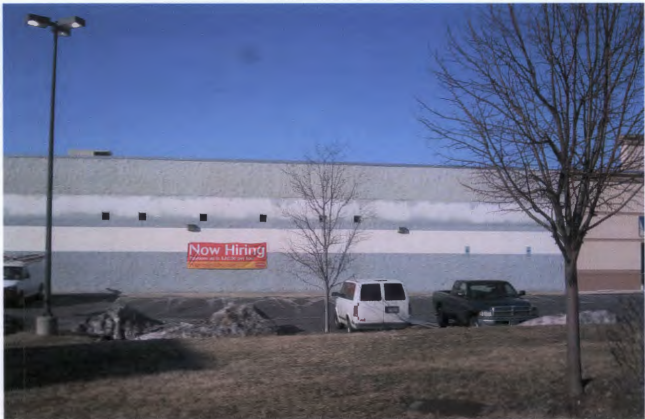
Baltimore National Pike side of building for HHGregg store
