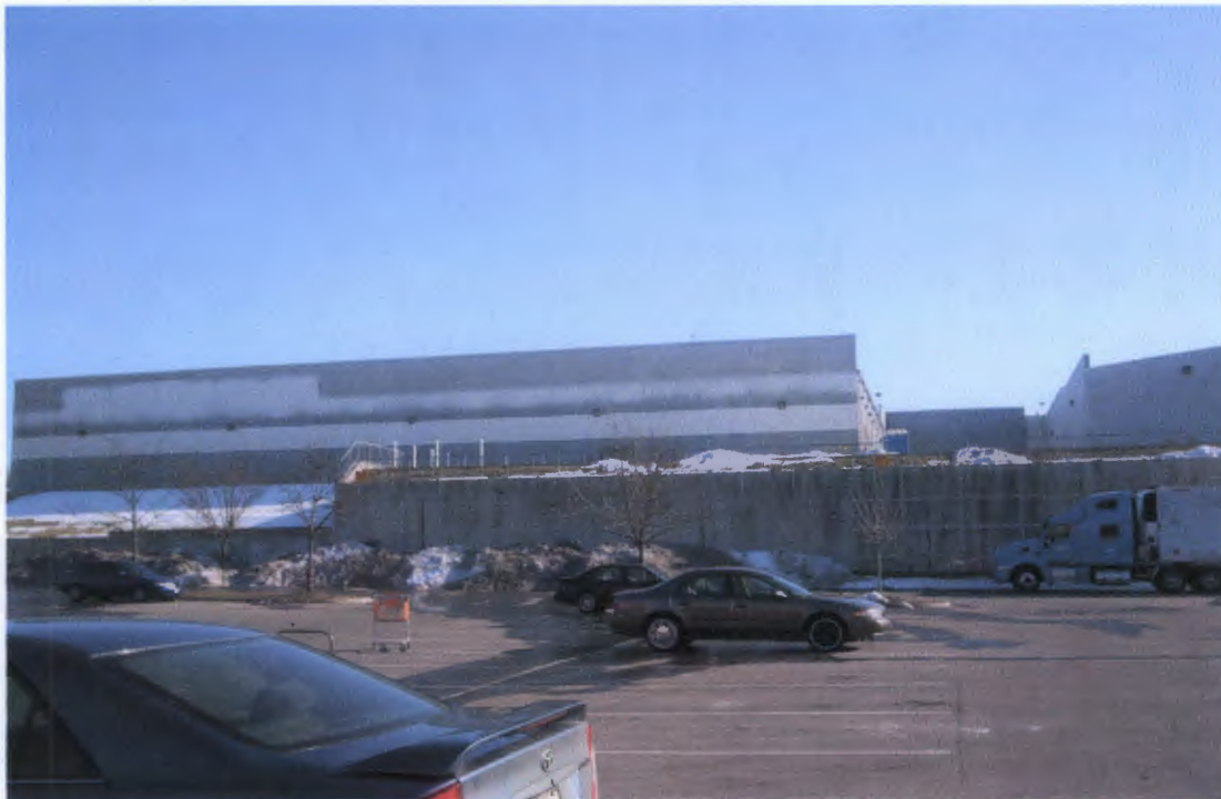
Rear of HHGregg store from Home Depot parking lot
