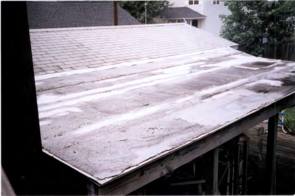
Shed and Deck to be razed.
