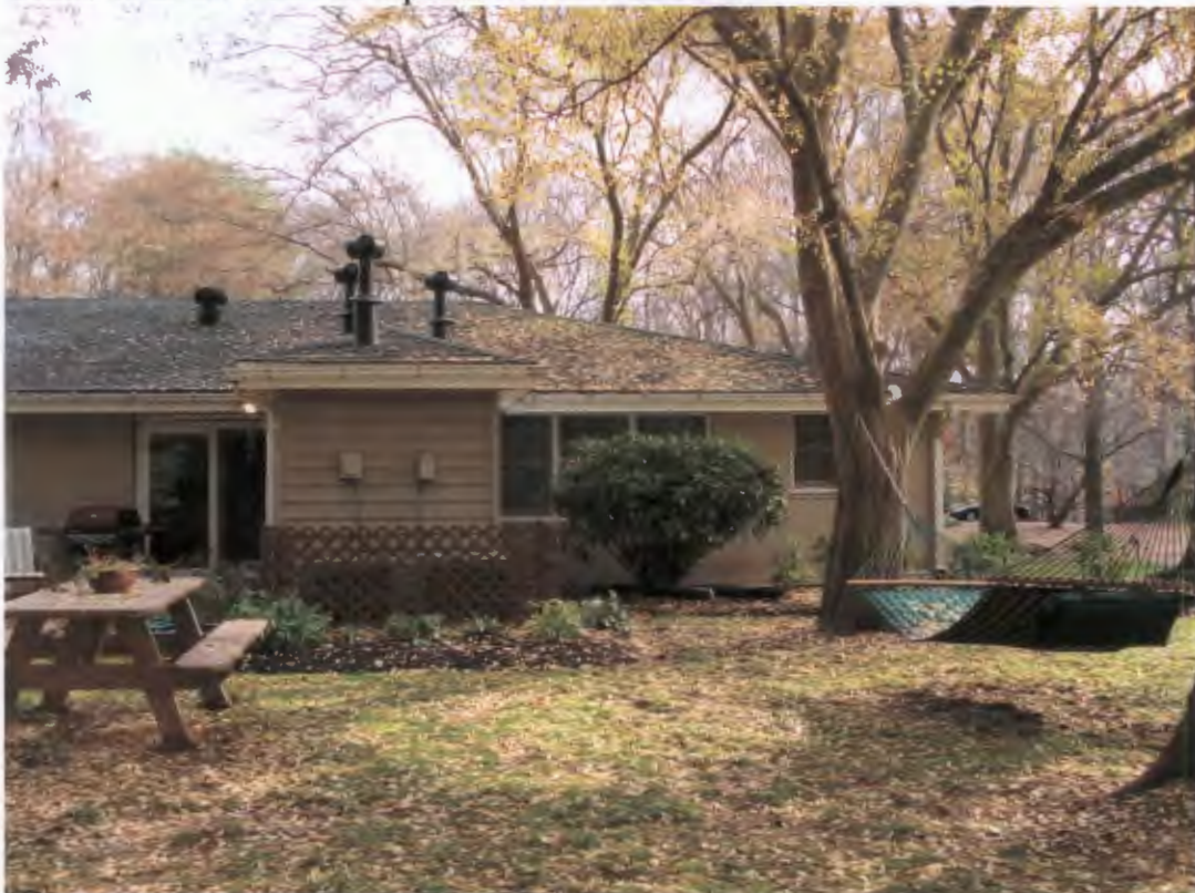
Master bath addition will be on the right side (rear picture) extending out.
