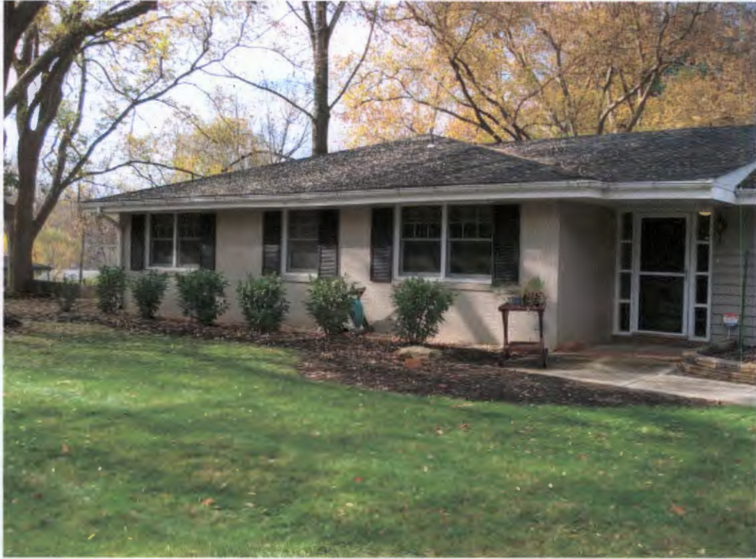
Front of where Master Bath addition (to left)
