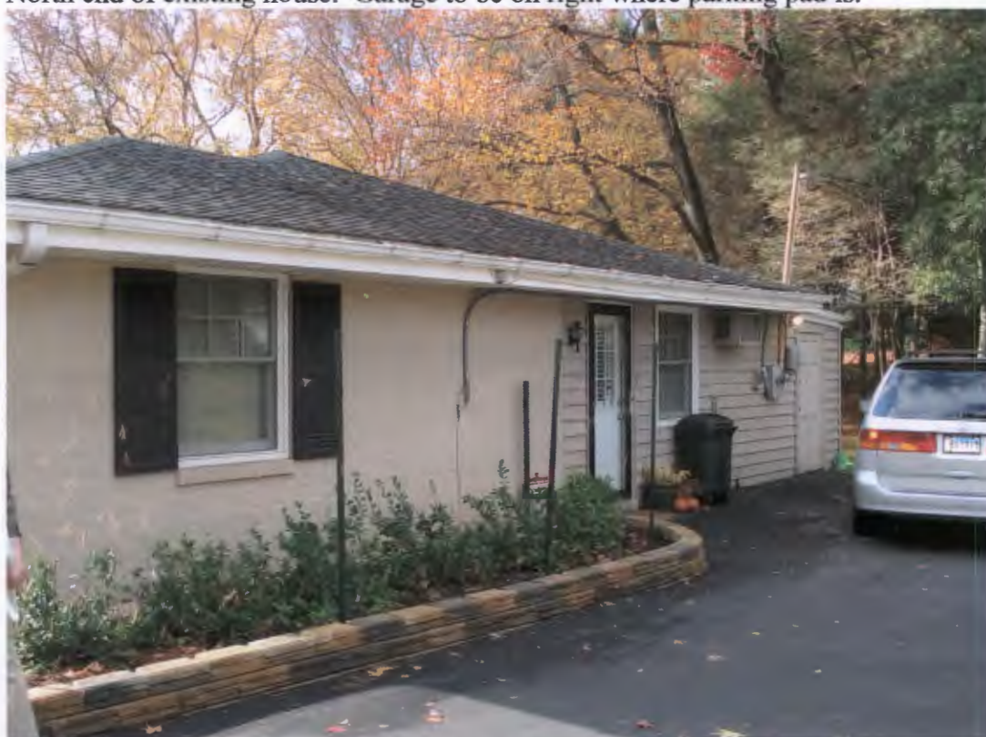
Side where garage is to go with access to side door for garage access.
