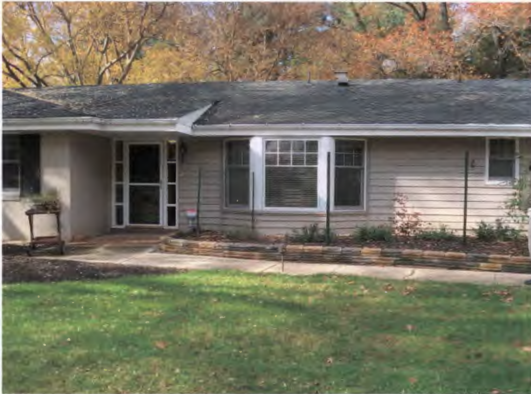
Center of house where new porch will be constructed.
