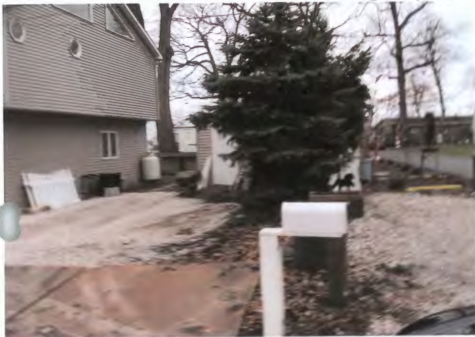
LOOKING FROM DRIVEWAY ENTRANCE TO WHERE PROPOSED GARAGE TO Be Built
