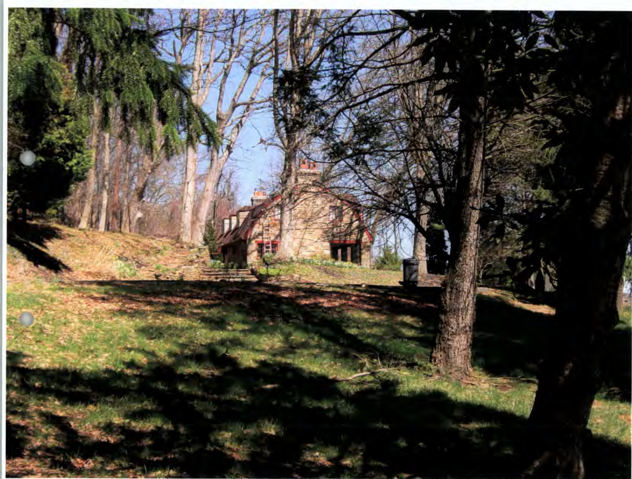
No 606 Hillstead Drive From "Common" Driveway
