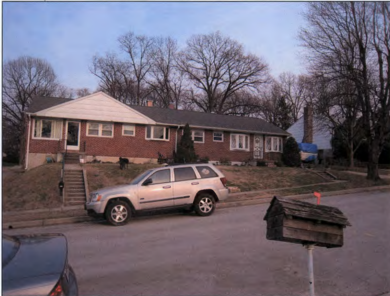
View of front of 5215 (left) and 5217 (right) Larlin Road taken from Larlin Road.
