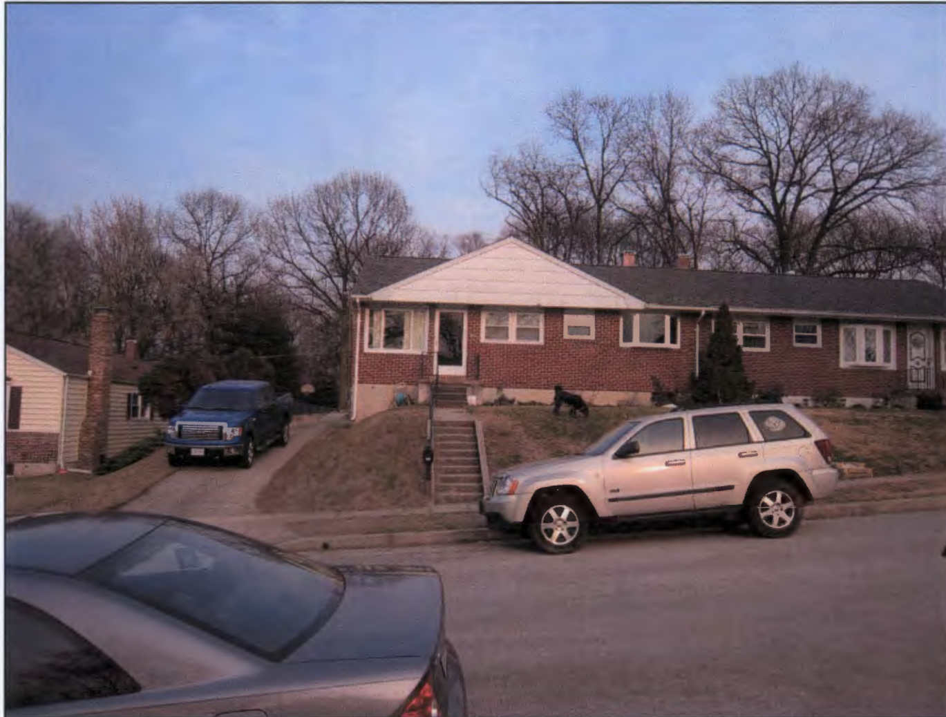
View of front of 5215 Larlin Road taken from Larlin Road.
