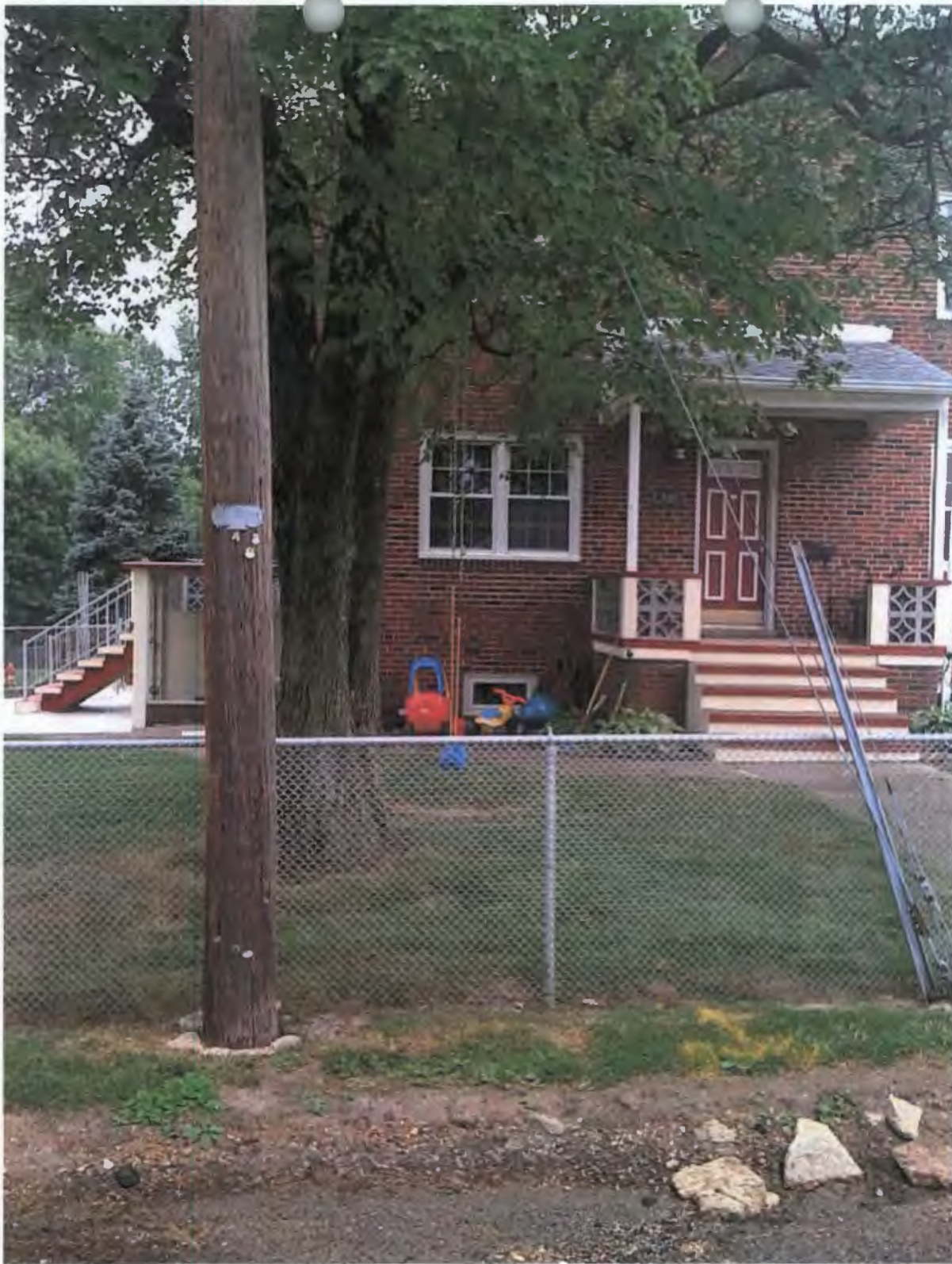
front view of 3105 Orchard Avenue
