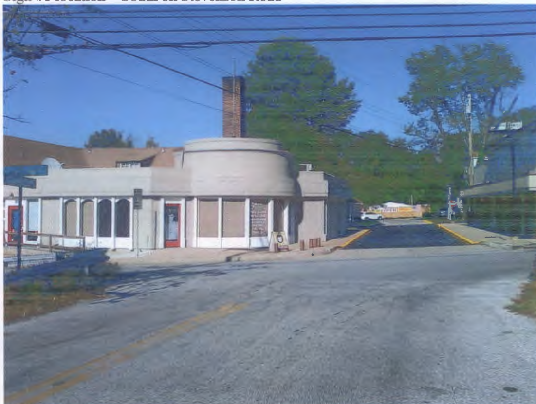
Sign #2 location – East on Old Valley Rd across Stevenson Road
