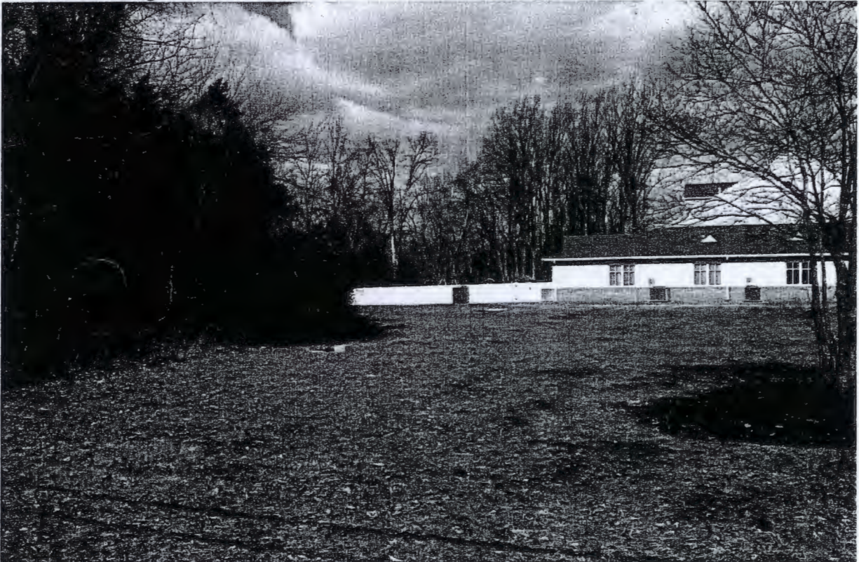
View from Windsor Mill Road. Building addition where fence is currently located.
