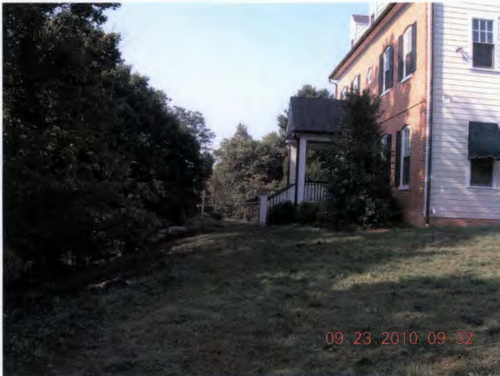
WESTERLY ALONG FRONT (MALVERN AVE.) ELEVATION
