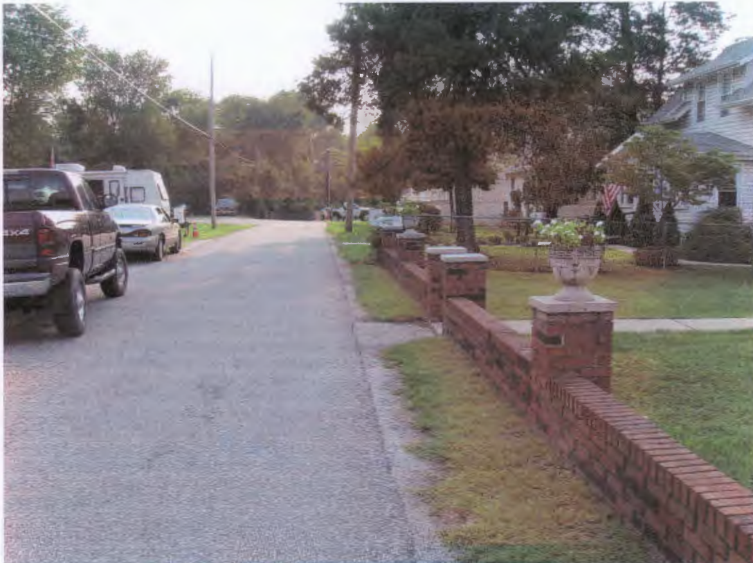
PENWOOD AVE LOOKING WEST
