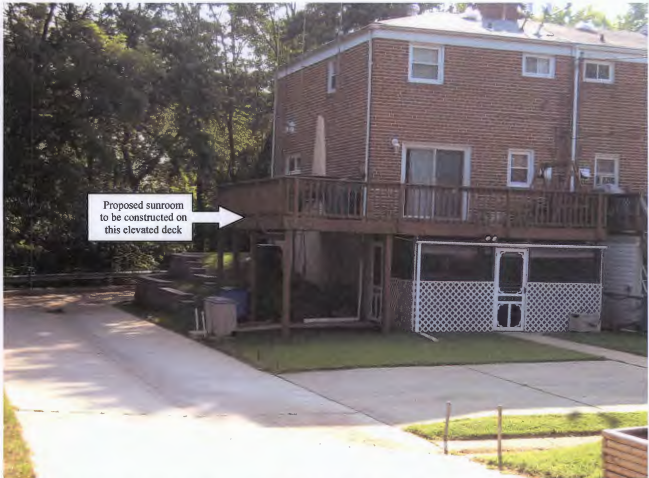
View of rear corner of dwelling and existing deck to be enclosed as seen from alley west of property
