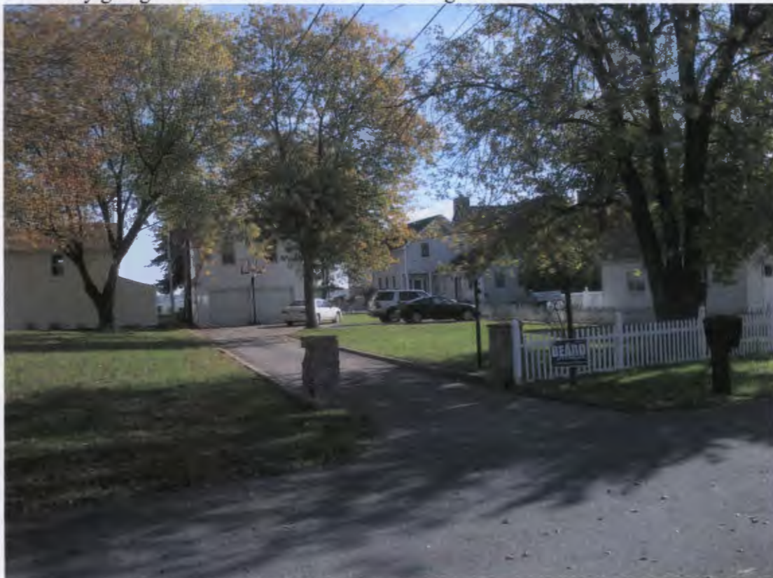
3709 Middle River Road garage and 3715 Middle River Road on left
