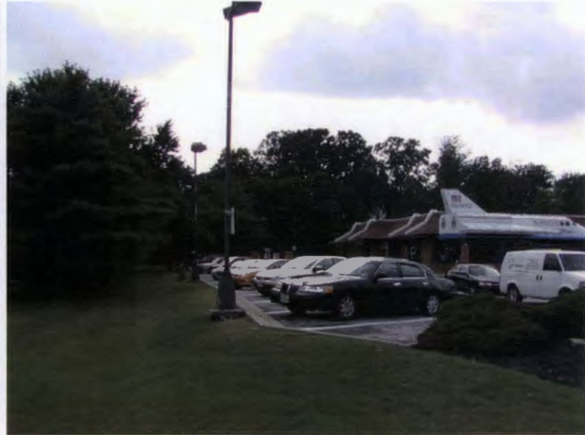
14- View South along East side of Ex. Building
