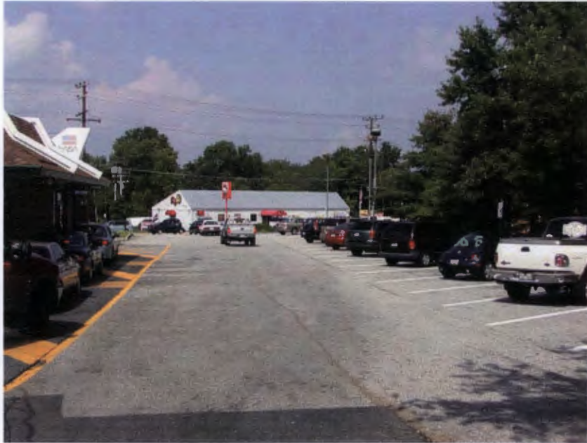
13- View along East side of Ex. Building toward Joppa Rd.
