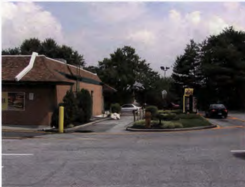
11- View East along Southside of Existing Building
