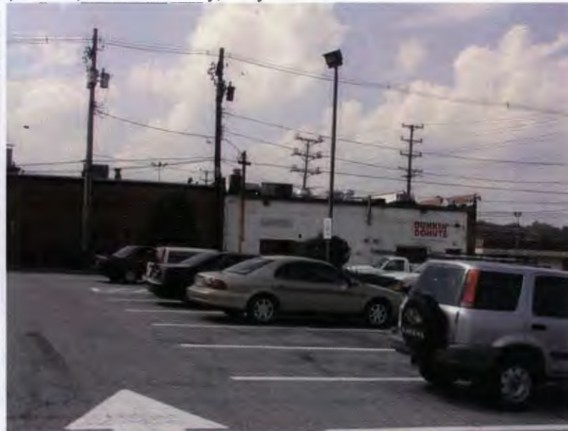
10- View along West side of Existing Building
