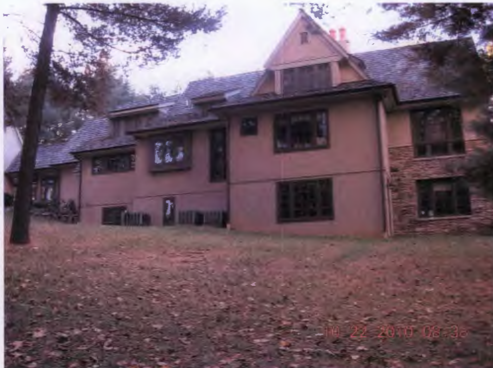
#14- NORTH ELEVATION OF EXISTING DWELLING
