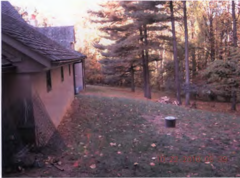
#15- LOOKING WESTERLY ALONG NORTH DWELLING ELEVATION
