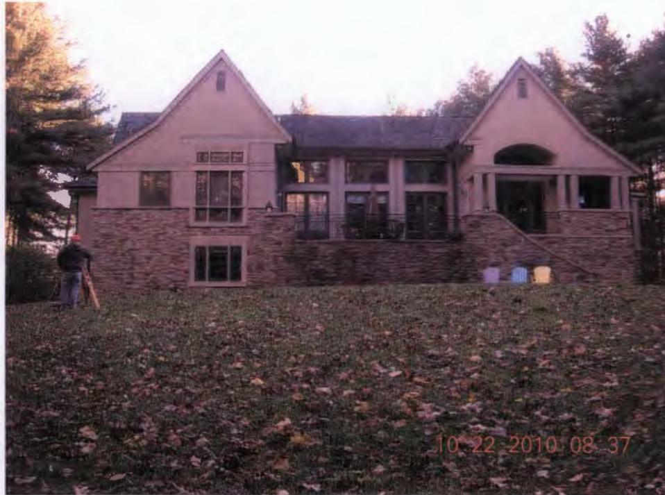
#9- REAR OF EXISTING DWELLING
