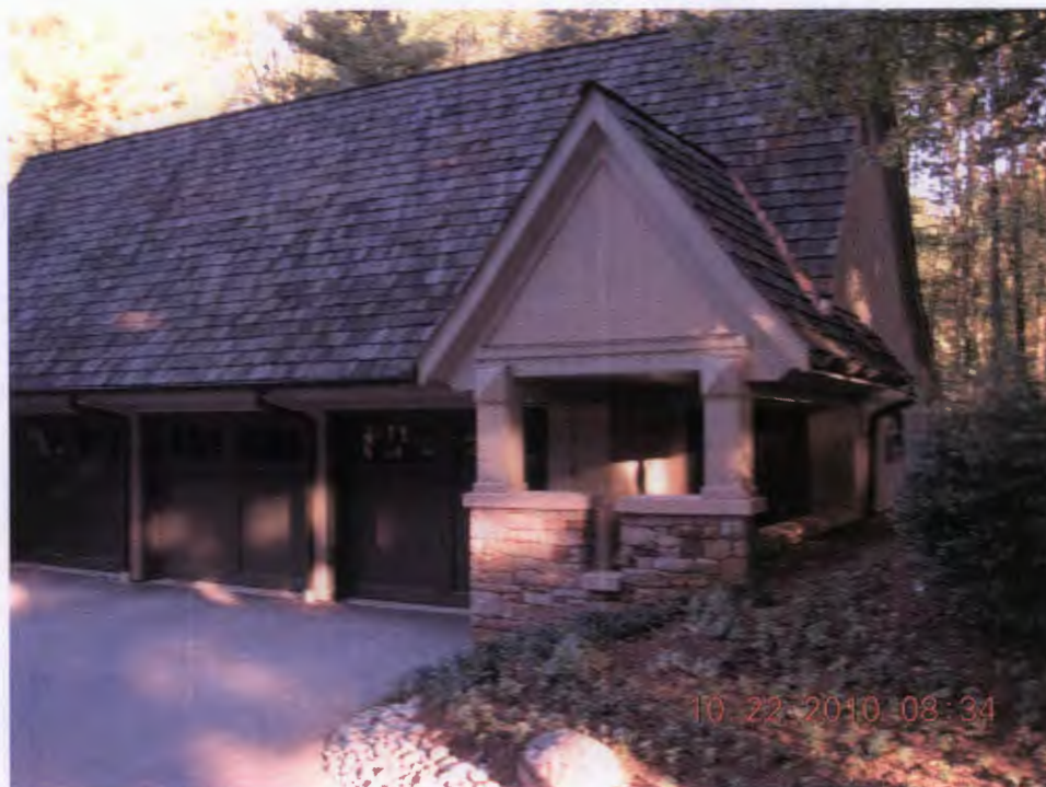
#6- FRONT OF EXISTING GARAGE
