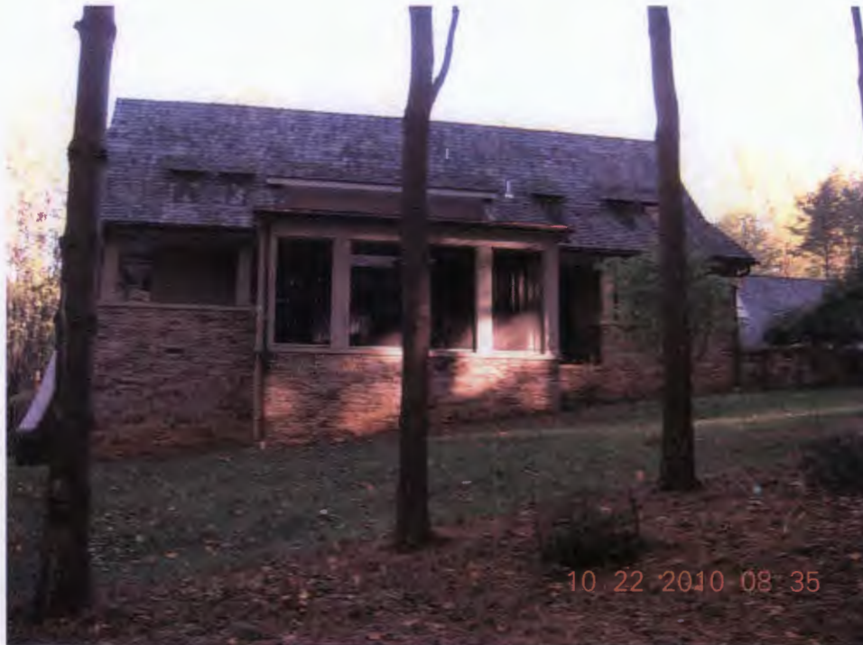
#7- SOUTH ELEVATION OF EXISTING DWELLING
