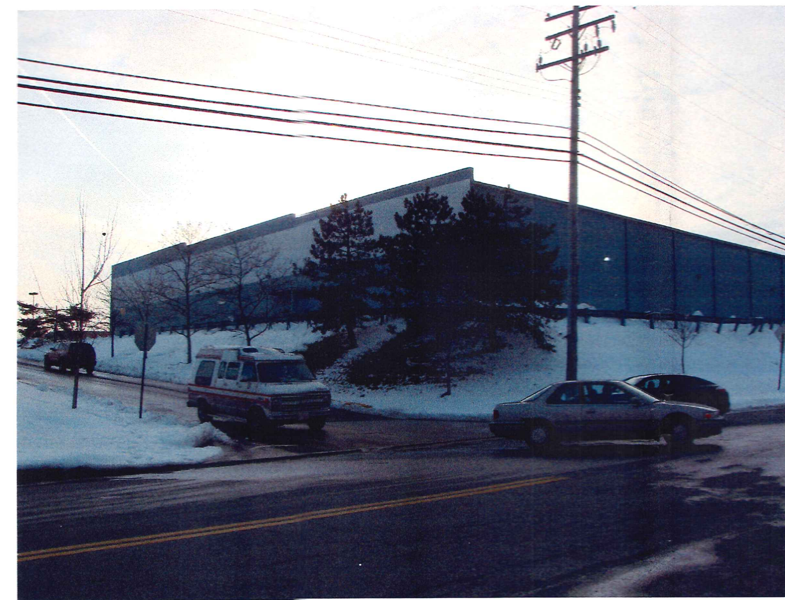
6- VIEW TO WEST AT NORTHERN ENTRY OF MOHRS LAND
