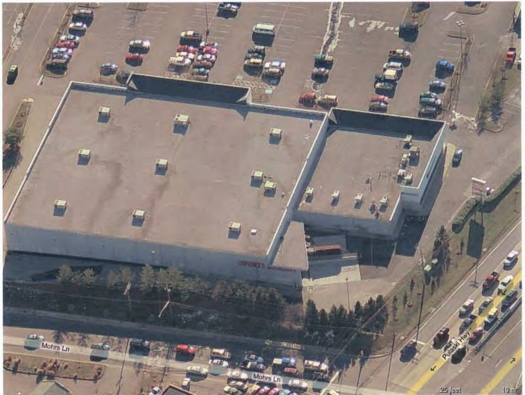
Birdseye View of Property Looking South
