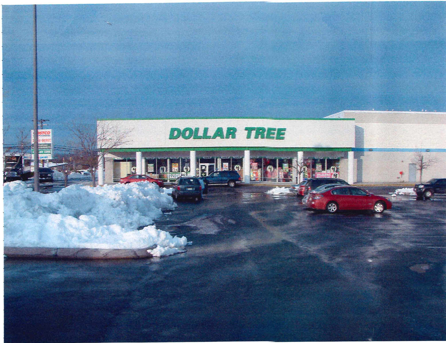
1- VIEW TO NORTH OF FRONT ENTRY FACADE
