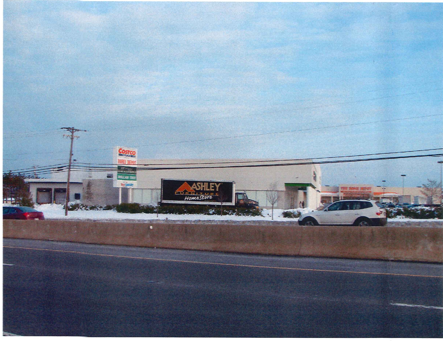
3- VIEW TO EAST FROM SOUTH BOUND SHOULDER OF PULASKI HIGHWAY
